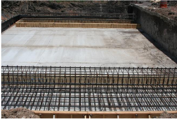
(a) Footing Reinforcement
