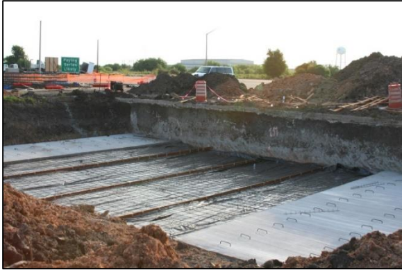
(a) Formwork and Reinforcement
