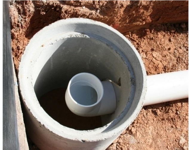
(b) Manhole Placement
