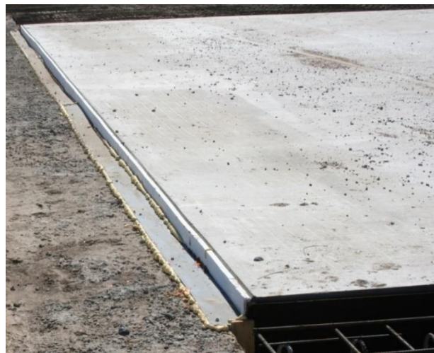
(a) Expansion Joint and Steel Sheet Form.
