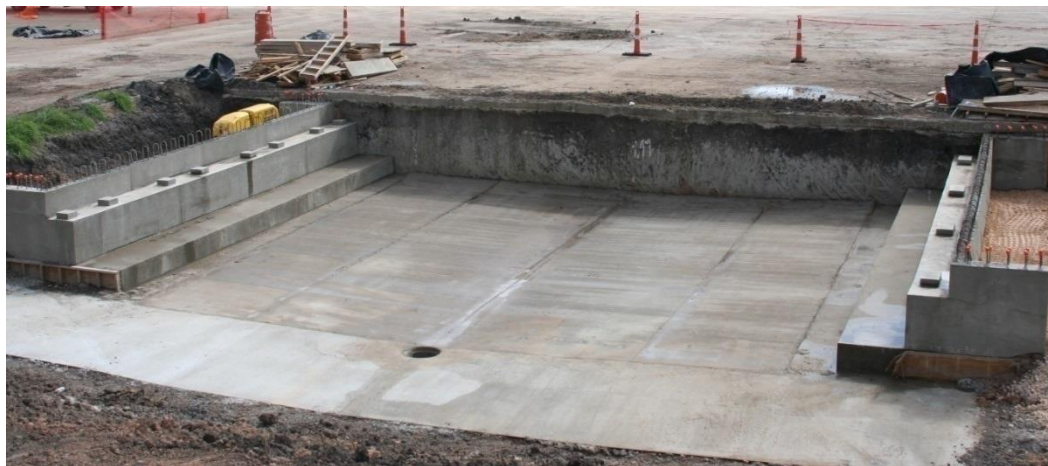
Figure 4.12. Substructure after Removal of the Forms.
