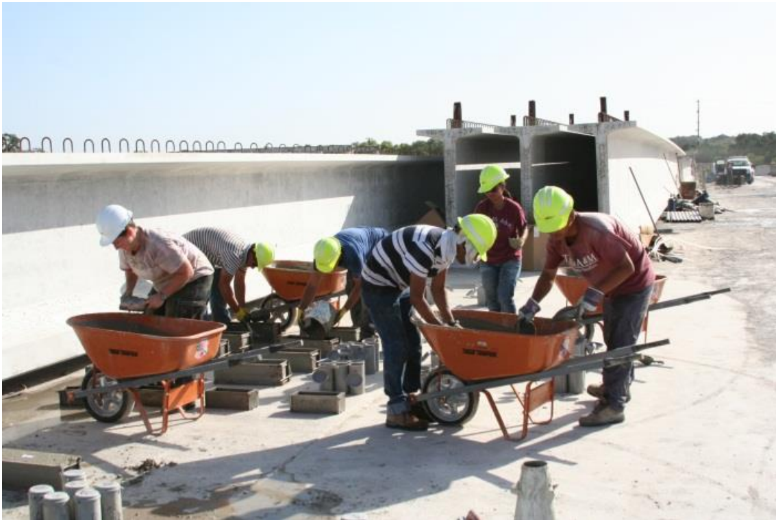
Figure B.30. Test Specimen Casting.
