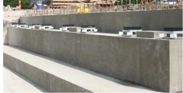
(b) South End Load Cell Assembly
