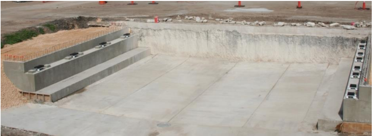
(c) Bridge Span Ready for Girder Placement
