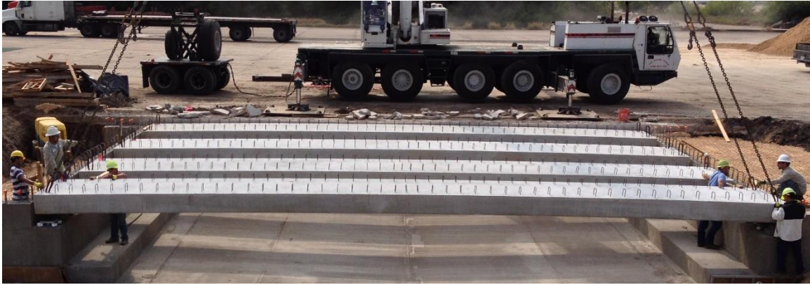
(a) Slab Beam Placement
