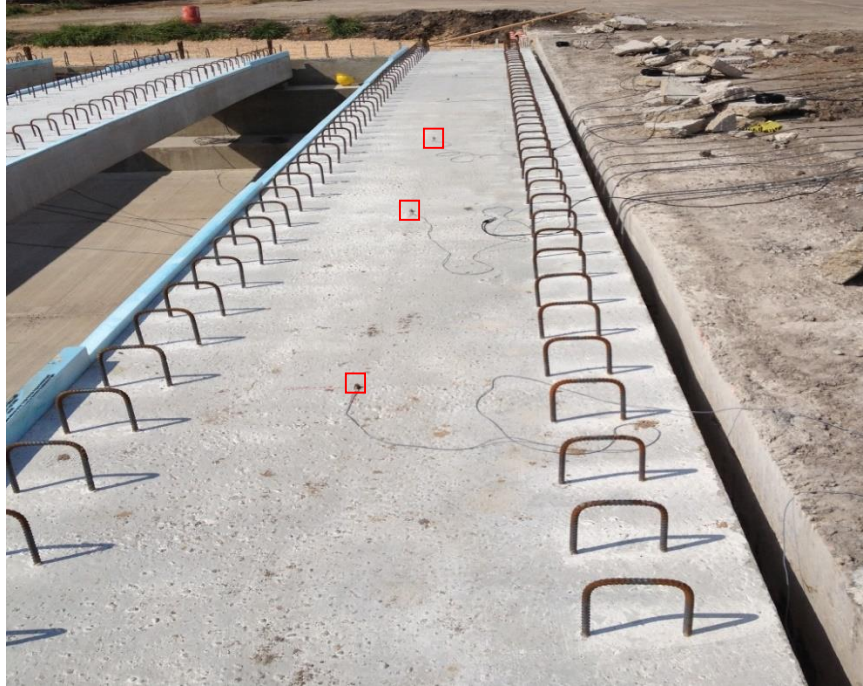
Figure 5.7. Accelerometer Positions for Individual Beam Test.
