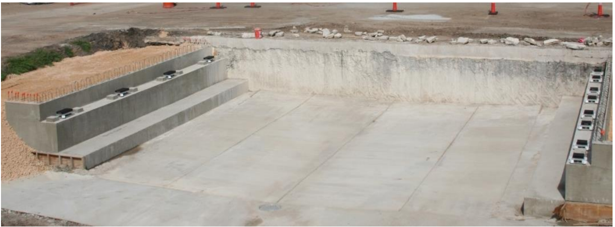
(c) Bridge Span Ready for Taking the Girders
