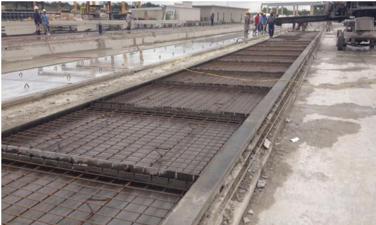
Figure B.18. Precast Concrete Panel Construction.
