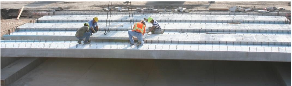
(c) Erection of Precast Concrete Panels
