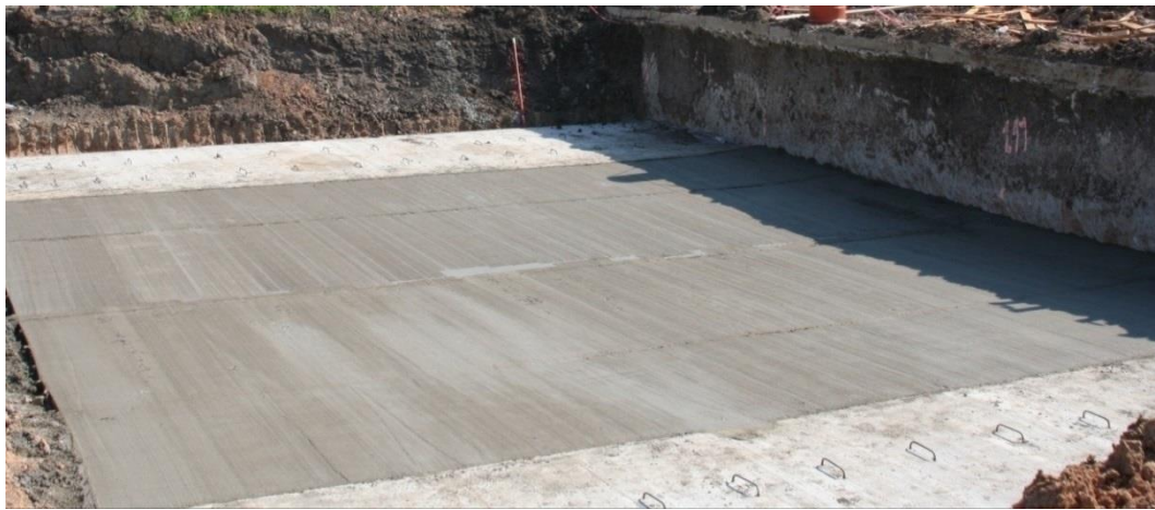
(c) View of Slab-on-Grade after Broom Finish
