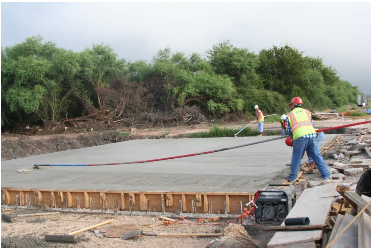
Figure B.22. Deck Concrete Finishing.
