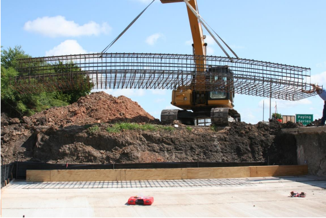
(a) Reinforcing Cage Placement
