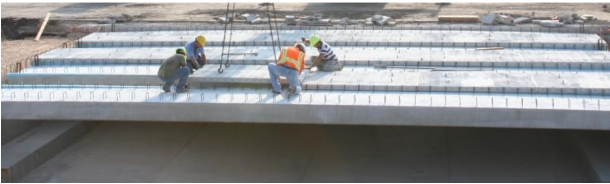
(b) Precast Panel Erection
