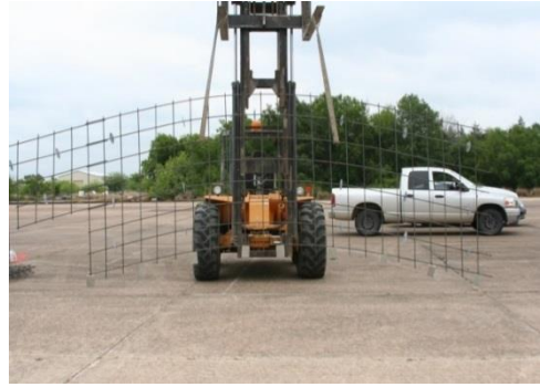
(b) Rebar Mesh Installation
