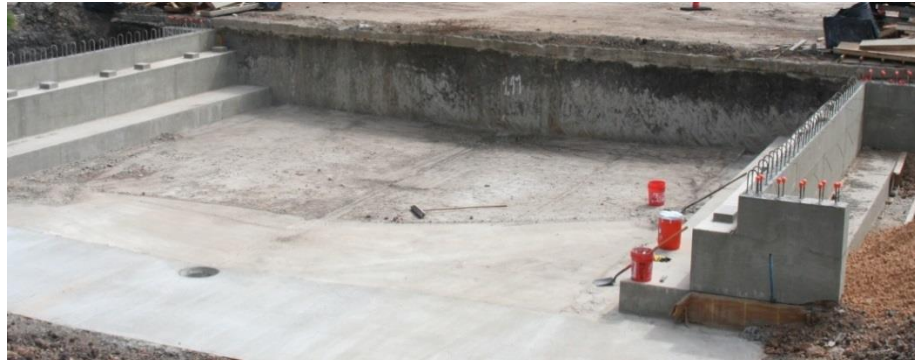
(b) View of the Substructure after Removal of the Forms
