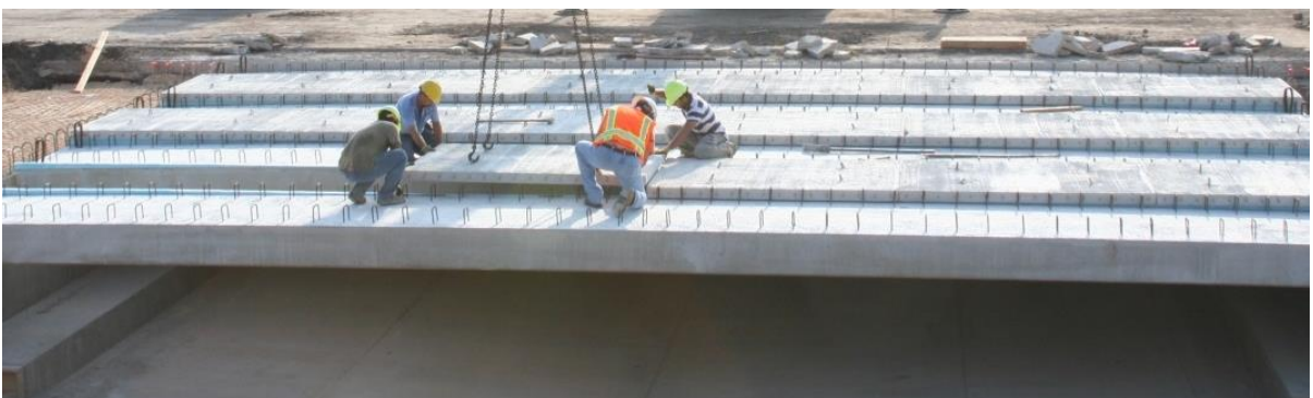
(c) Placement of Precast Concrete Panels
