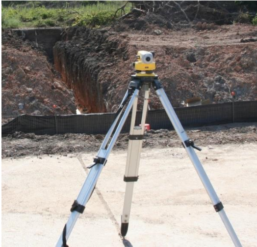
(a) Trench Excavation
