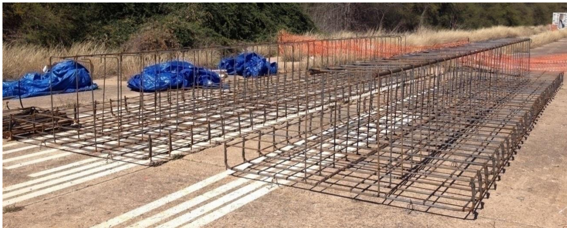
Figure B.12. Footing and Abutment Reinforcement Cage.
