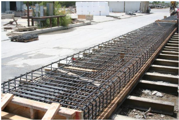
(a) Slab Beam Reinforcement
