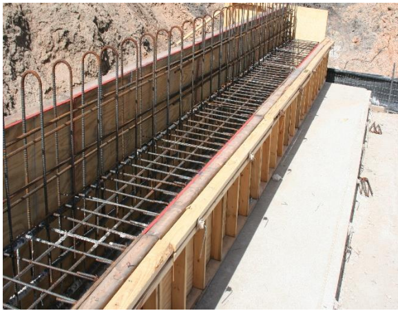
(c) Abutment Reinforcement
