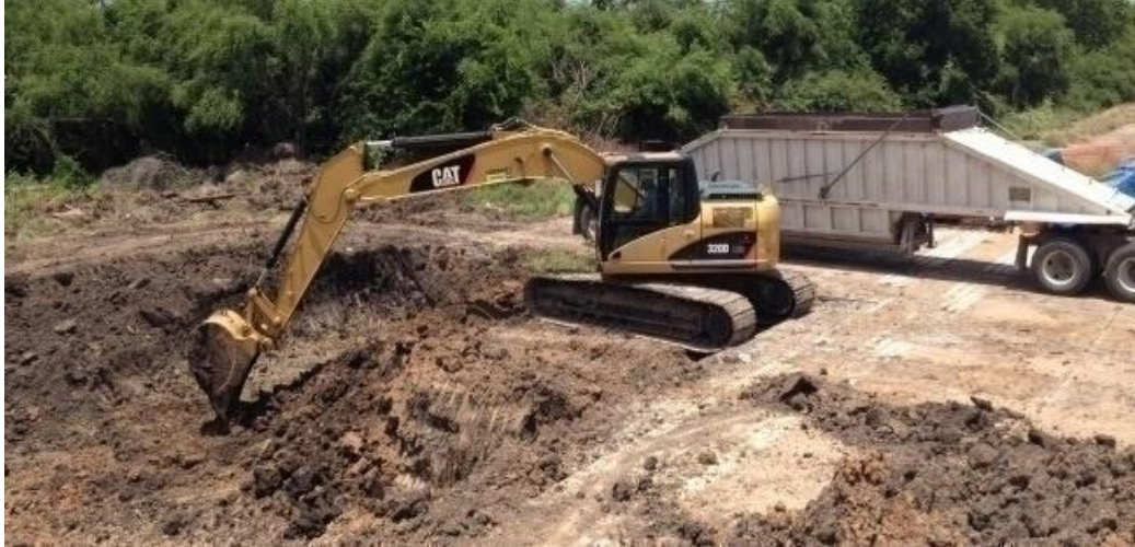
(a) Main Excavation of the Bridge Foundation
