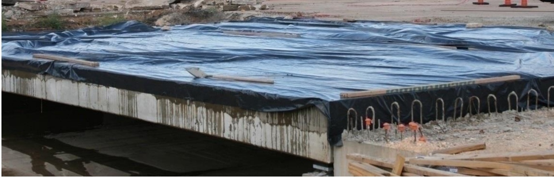
Figure B.23. Curing of Deck Concrete.
