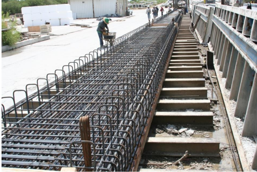
(a) Slab Beam Reinforcing Bar Placement
