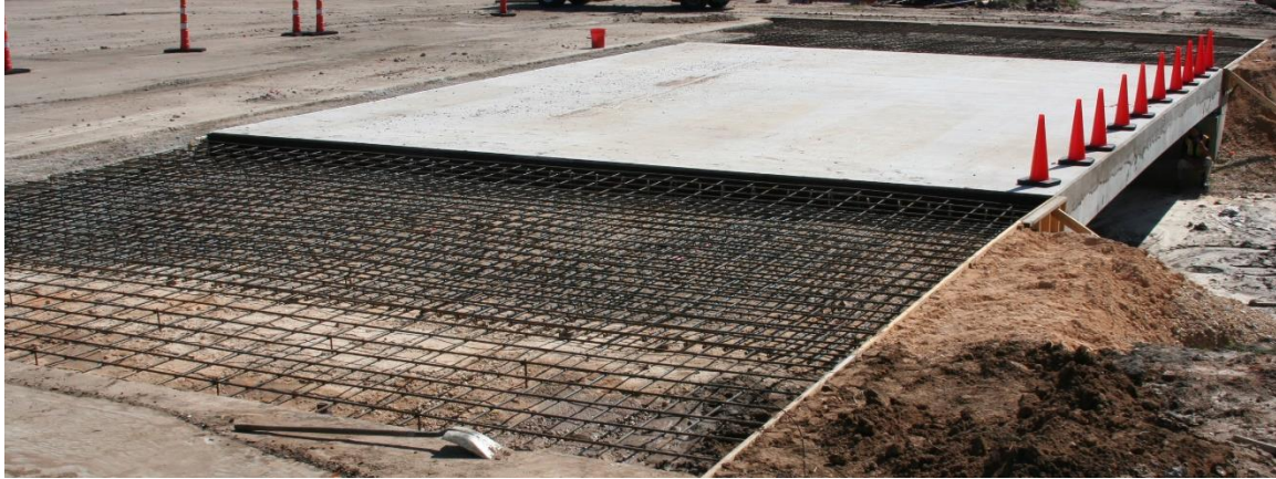
(a) Approach Slab Reinforcement
