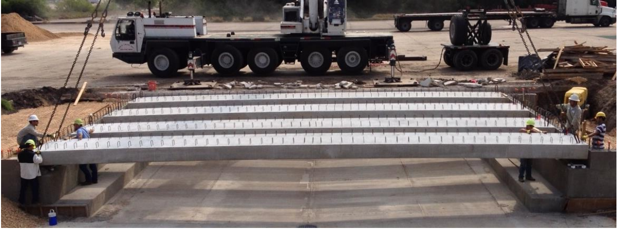
(a) Slab Beam Erection Operation
