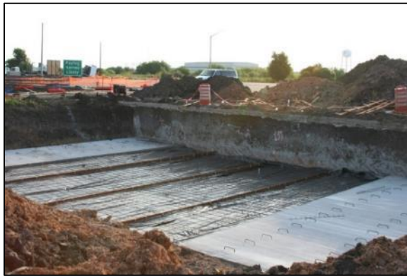
(a) Formwork and Reinforcement
