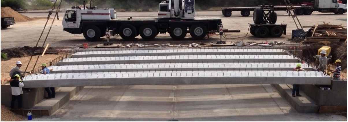
(a) Slab Beam Placement
