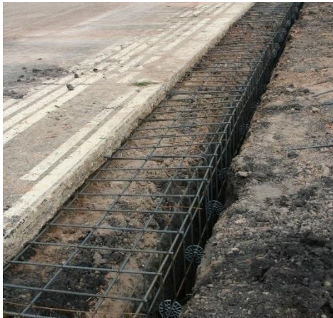
(a) Retaining wall Reinforcing Mesh
