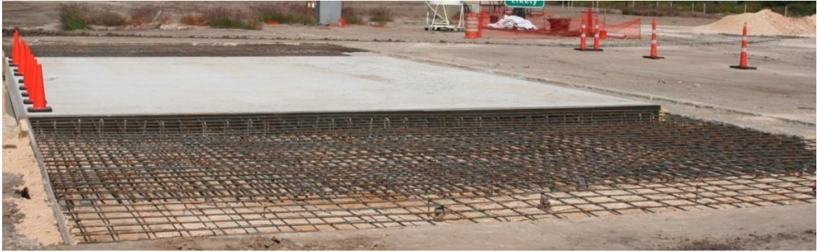
(b) Approach Slab Reinforcing Mesh
