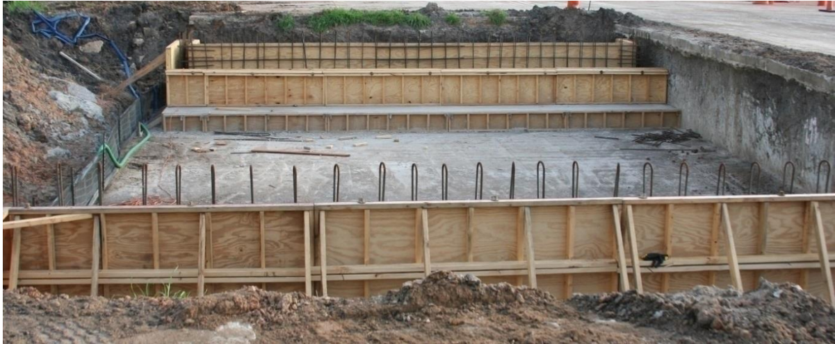
(a) Abutment and Wing-Wall Formwork Construction
