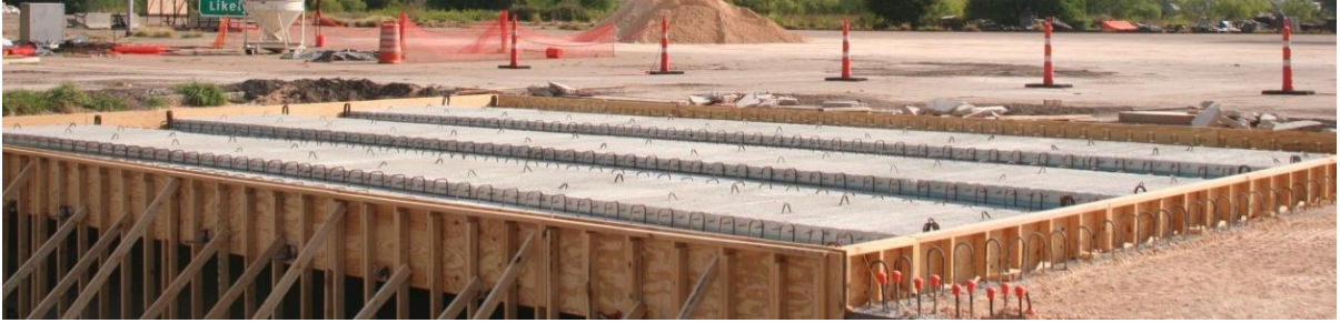
(a) Deck Formwork Construction
