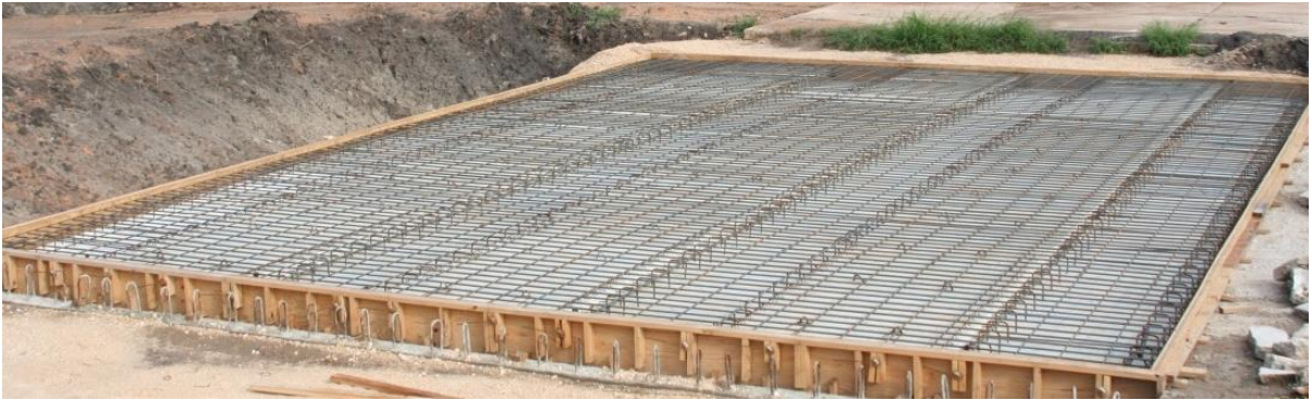
(b) Deck Reinforcing Bar Construction
