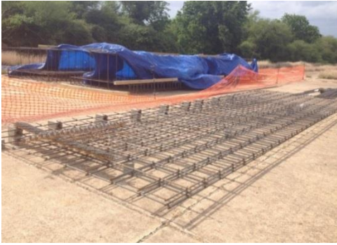
(a) Rebar Tying
