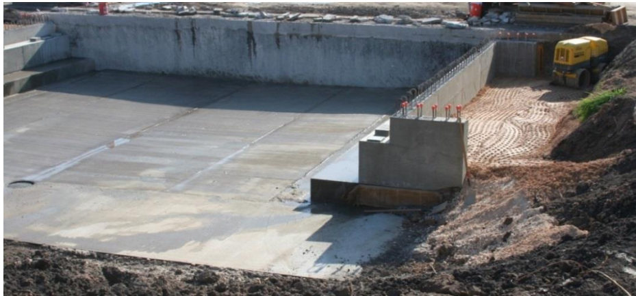
(c) Backfilling and Compaction Process
