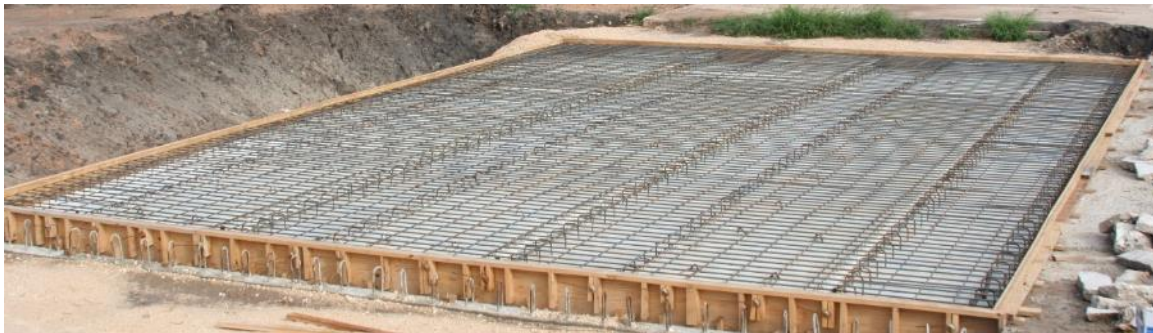
(a) Deck Reinforcement
