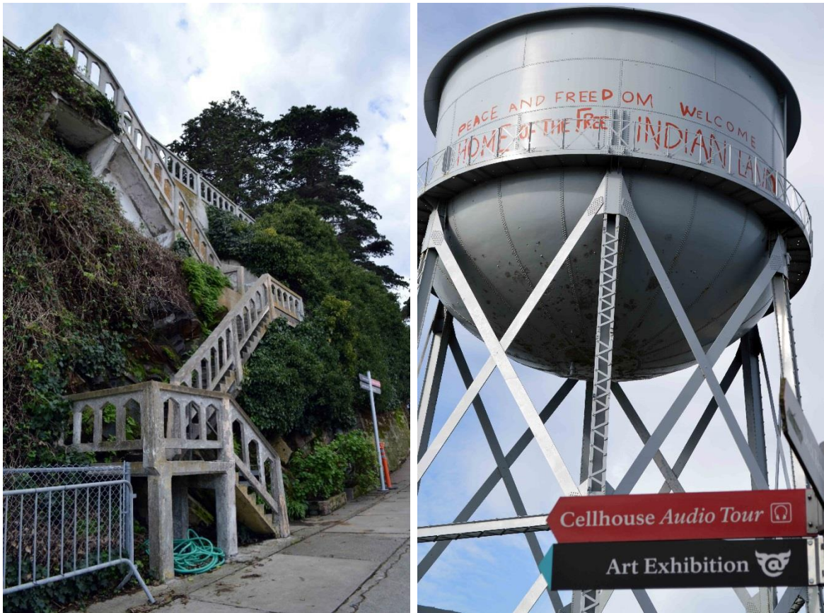
Figure 4 (a) Puppy Stairs; (b) Water Tower Graffiti (Manrique 2014)
