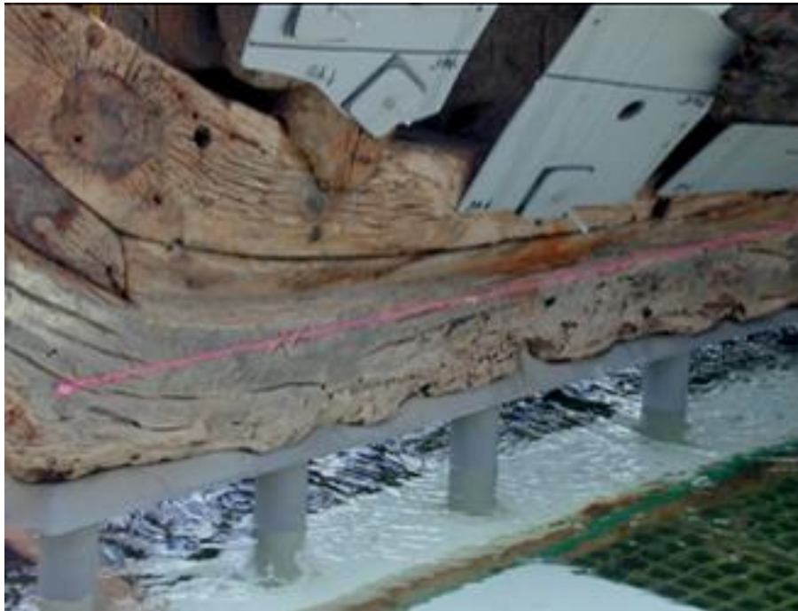
Figure 10.20. The finished keel plate at the bow illustrating the extent that the keel plate needed to rise in order to match the undulating deterioration on the bottom of the keel. Photo courtesy Conservation Research Laboratory and the Texas Historical Commission.
