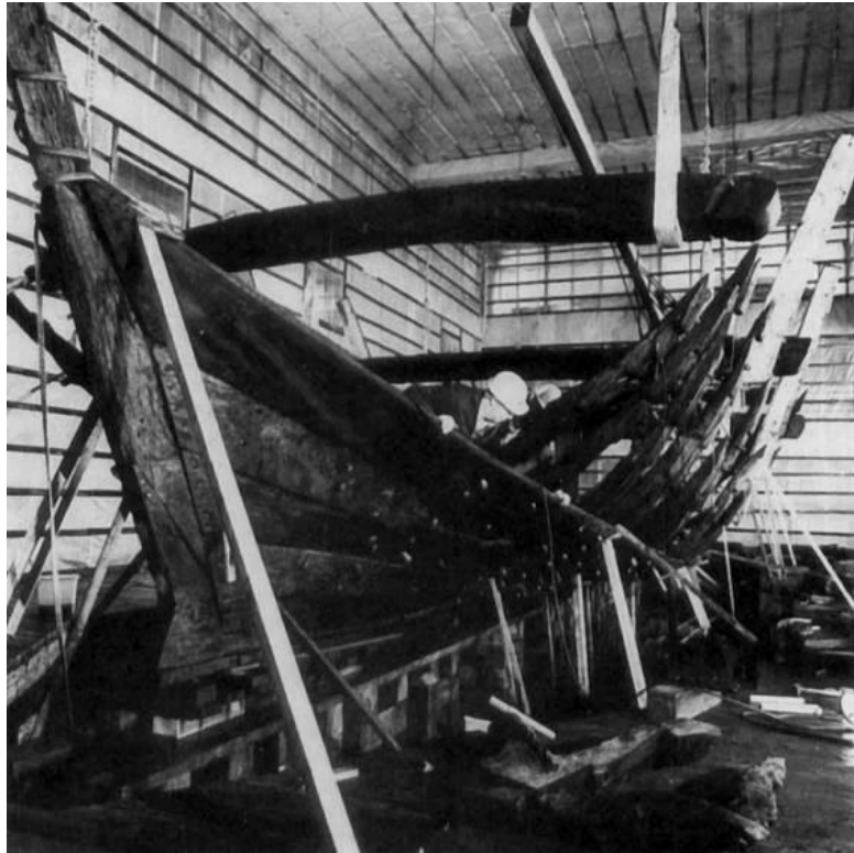
Figure 9.2. The reconstruction of the Bremen cog during the 1970s. Note the keel blocks under the sternpost lower left corner of the image. From Hoffmann 1986, 216.
