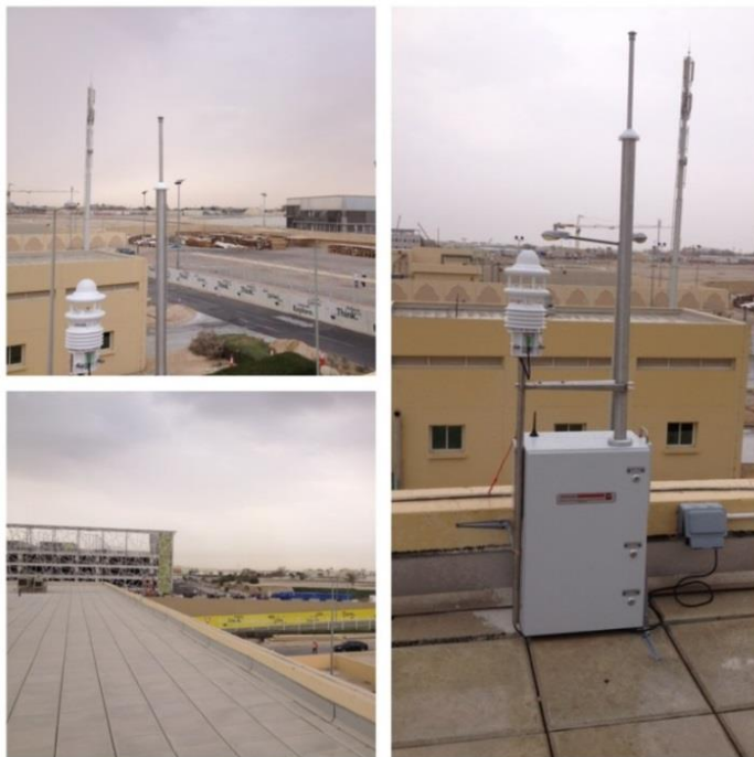
Figure 4 Monitoring station installed on a building rooftop at a background location
