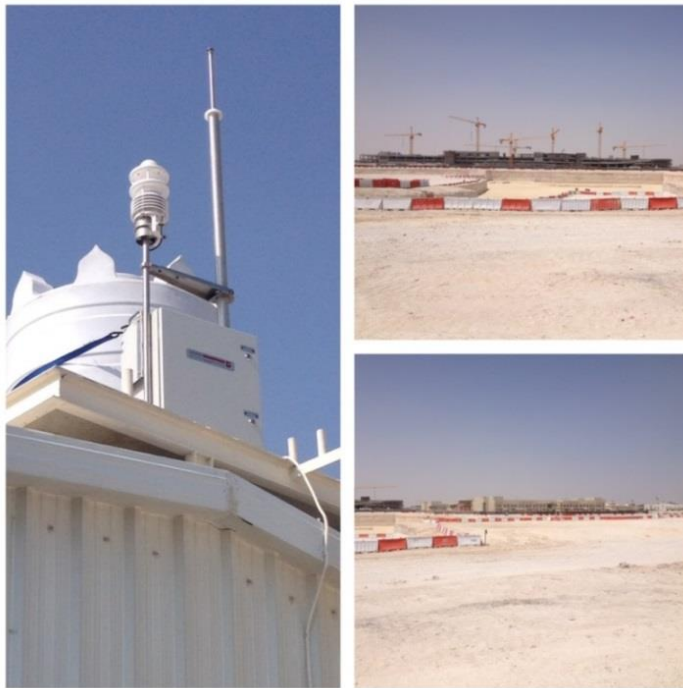
Figure 3 Monitoring station installed at a construction site at rest
