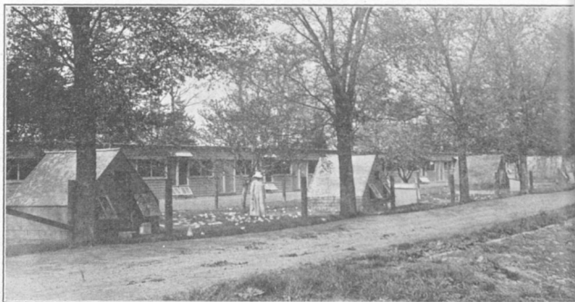
Fig. 18—A row of colony houses at the Old Cornell University Poultry Plant. The plant has since been moved to a less congested location.
