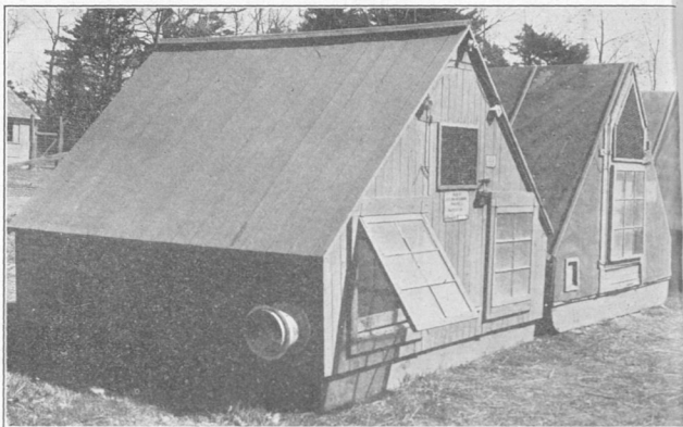
Fig. 17—Movable A-shaped colony house and method of coupling together for winter use. This type of house is too hot in the summer in Texas climate. The sides should be hinged to swing out and up. Too much glass in front for Texas climate.
