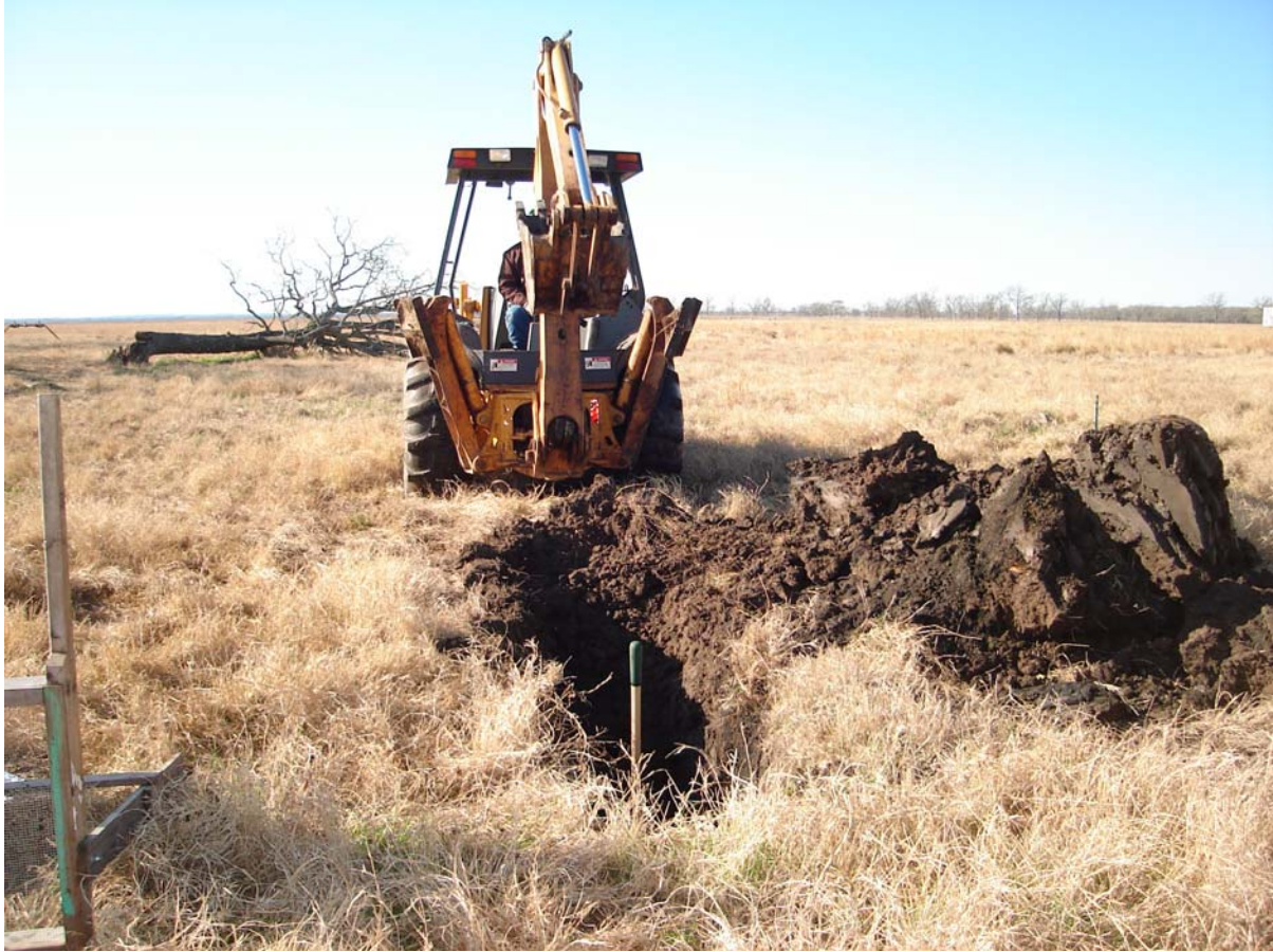
Figure 7. Backhoe Trench 2 (A-1 Well)
