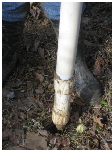
Figure 4. Picture of the well being placed into the excavated area
