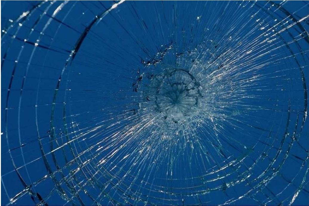
Figure 47: Photograph of Glass Fracture Depicting Concentric Cracks
