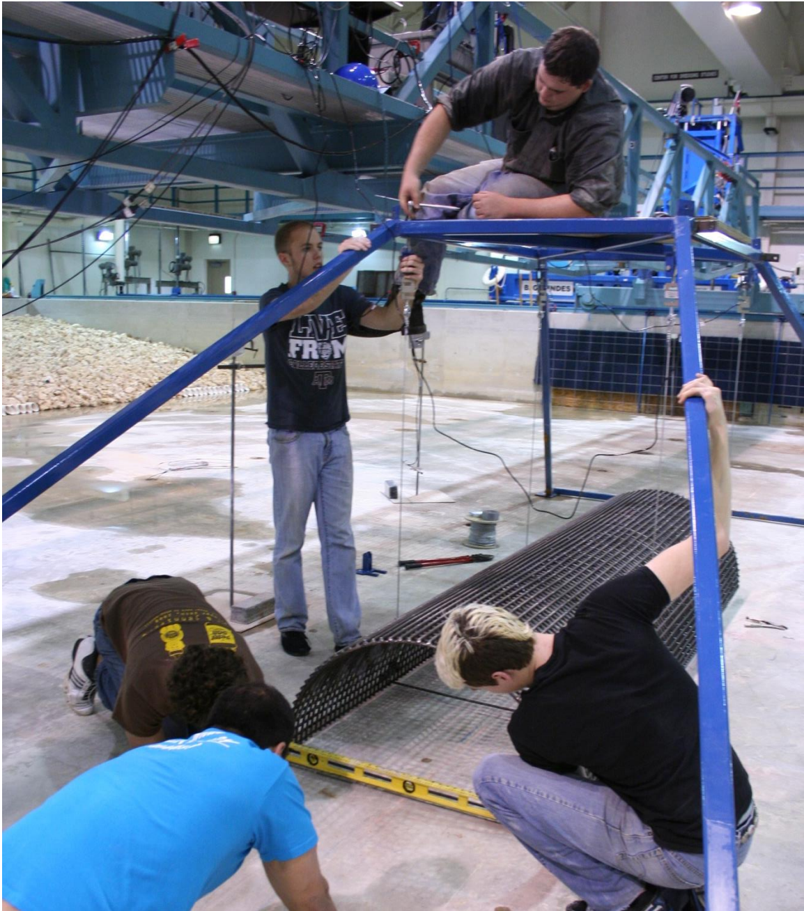
Figure 54. Installation of the breakwater (setting floor clearance)
