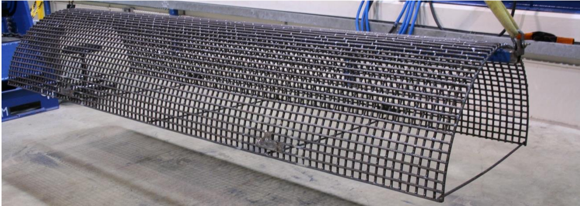
Figure 5. Complete submerged breakwater structure.
