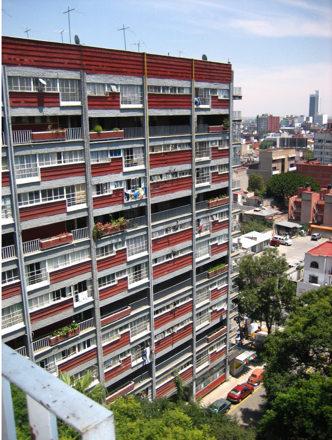
Figure 29. Building Selected for the Energy Simulation from the Multifamiliar Miguel Aleman at the Corner of Felix Cuevas Avenue and Coyoacan Avenue (South-SouthWest Façade) (Photo by Jose Luis Bermudez Alcocer).
