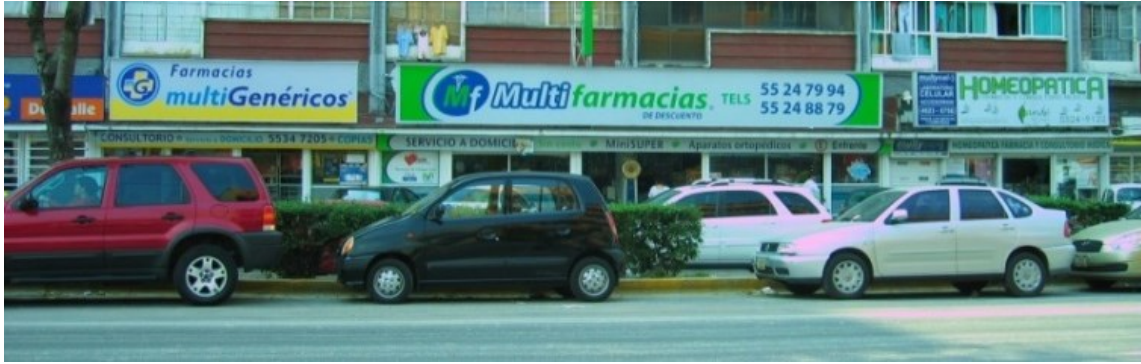
Figure 62. First Floor of the Building Analyzed: Part 2 (Photo by Jose Luis Bermudez Alcocer).
