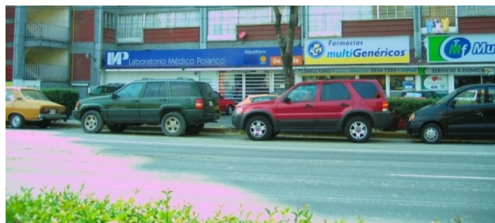
Figure 61. First Floor of the Building Analyzed: Part 1 (Photo by Jose Luis Bermudez Alcocer).
