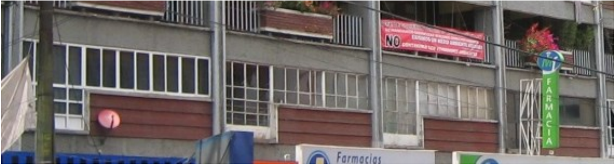
Figure 41. Single-Glass Window on East-SouthEast Façade. (Photo by Jose Luis Bermudez Alcocer).
