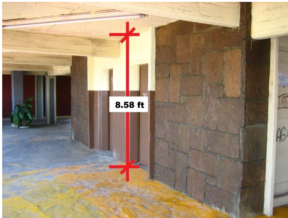
Figure 38. Detail to Calculate Height Floor-to-Ceiling for the Apartments (Photo by Jose Luis Bermudez Alcocer).
