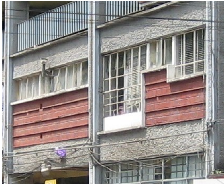
Figure 42. Single-Glass Window on South-SouthWest Façade. (Photo by Jose Luis Bermudez Alcocer).
