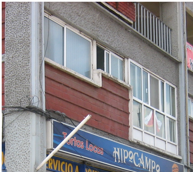
Figure 40. Single-Glass Window on North-NorthEast Façade. (Photo by Jose Luis Bermudez Alcocer).
