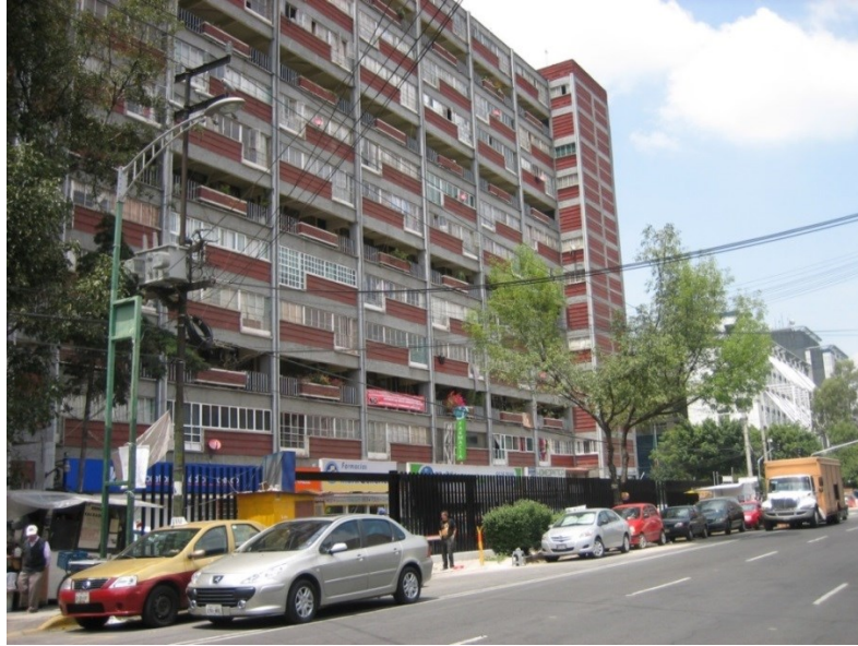
Figure 27. Building Selected for the Energy Simulation from the Multifamiliar Miguel Aleman at the Corner of Felix Cuevas Avenue and Coyoacan Avenue (East-SouthEast Façade) (Photo by Jose Luis Bermudez Alcocer).
