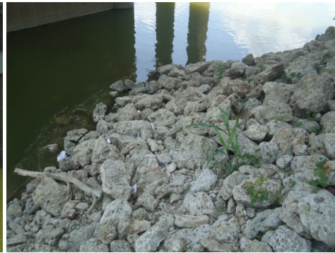
b. Riprap on the west side of the bridge
