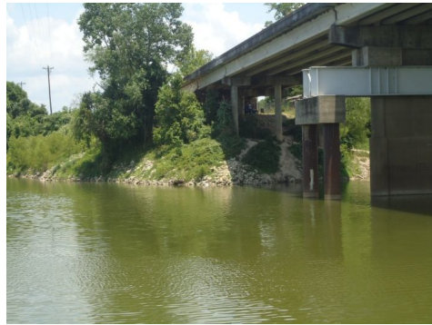
a. Riprap on the east side of the bridge
