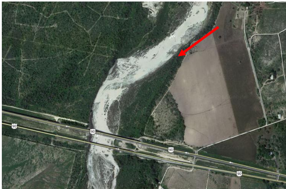
Figure 19. US 90 at Nueces River (Google Earth, 2013)
