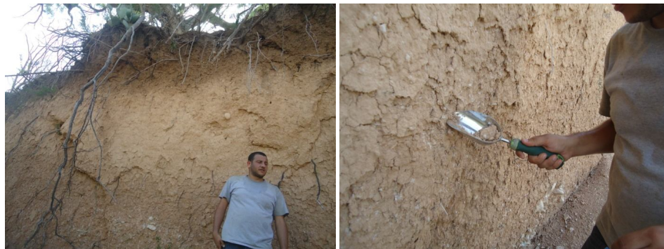
a. Erosion next to a tree
