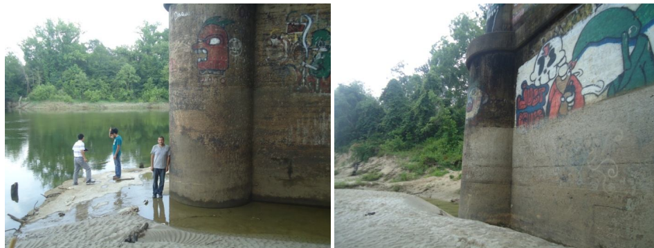
Figure 54. Column of the bridge
