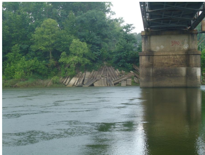
Figure 56. Concrete blocks at east side of bridge
