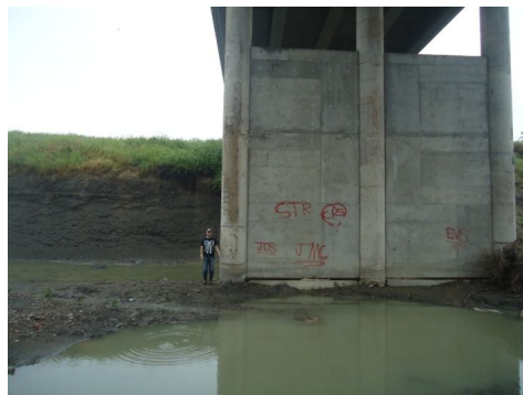
c. Column of the bridge
