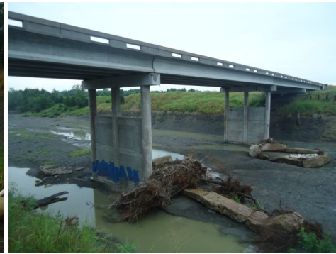
b. Bridge at SH 34
