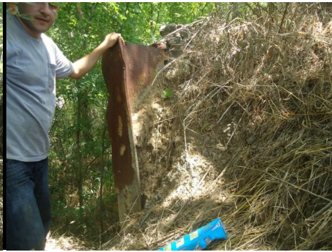
d. Old sheet pile
