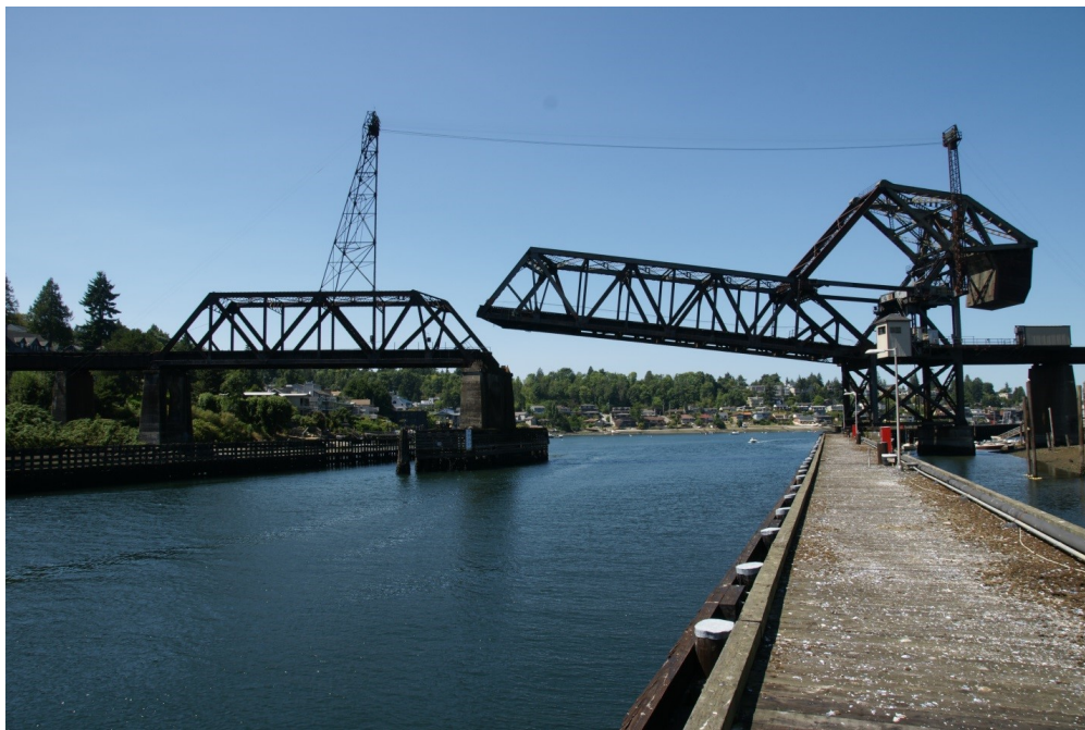
Figure 2.1: The Salmon Bay Bridge is a heel-trunnion bascule bridge in Seattle, WA. (Photo taken by Dr. Gary Fry.)
