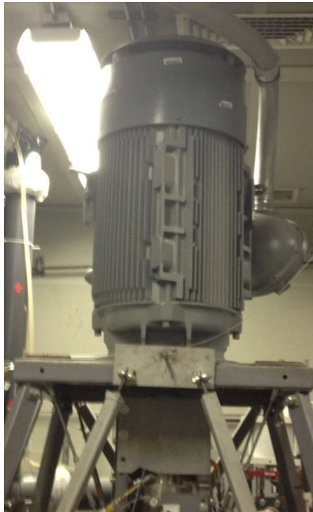
Figure 41. Motor Located at Top of Derrick
