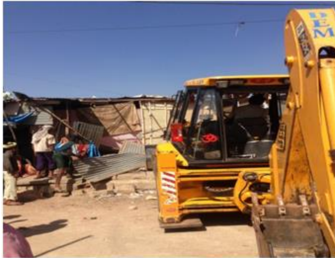
Figure 53. Bulldozers razing the tin sheds in Rajendranagar
