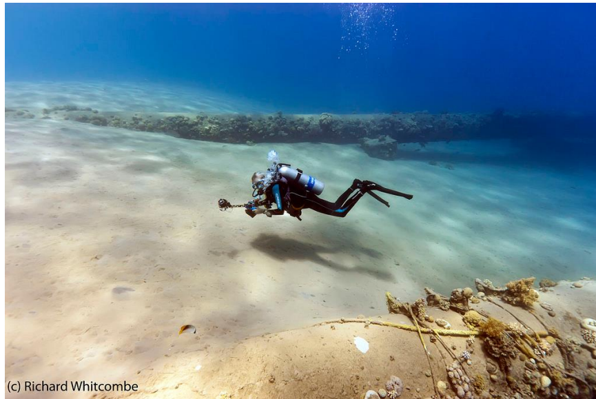
Fig. 1.2 An example of a free spanning pipeline with moderate marine growth (courtesy of Richard Whitcombe).
