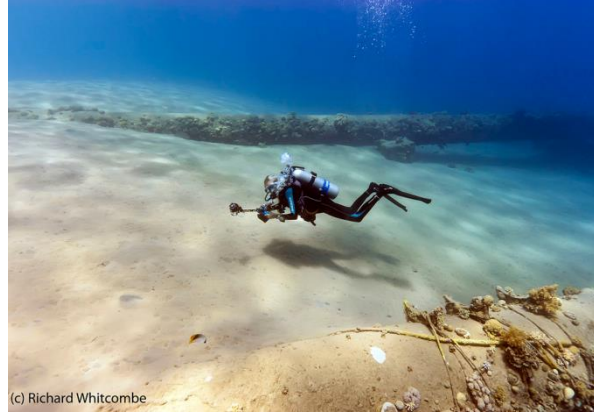
(d) Light marine growth of a free-spanning pipeline (courtesy of Richard Whitcombe)
