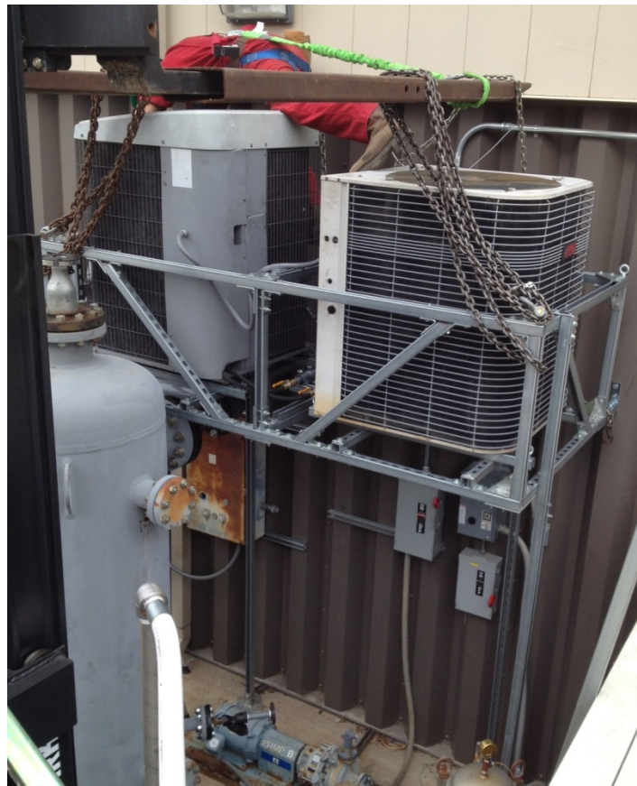
Figure 28: Installation of heat exchanger support structure
