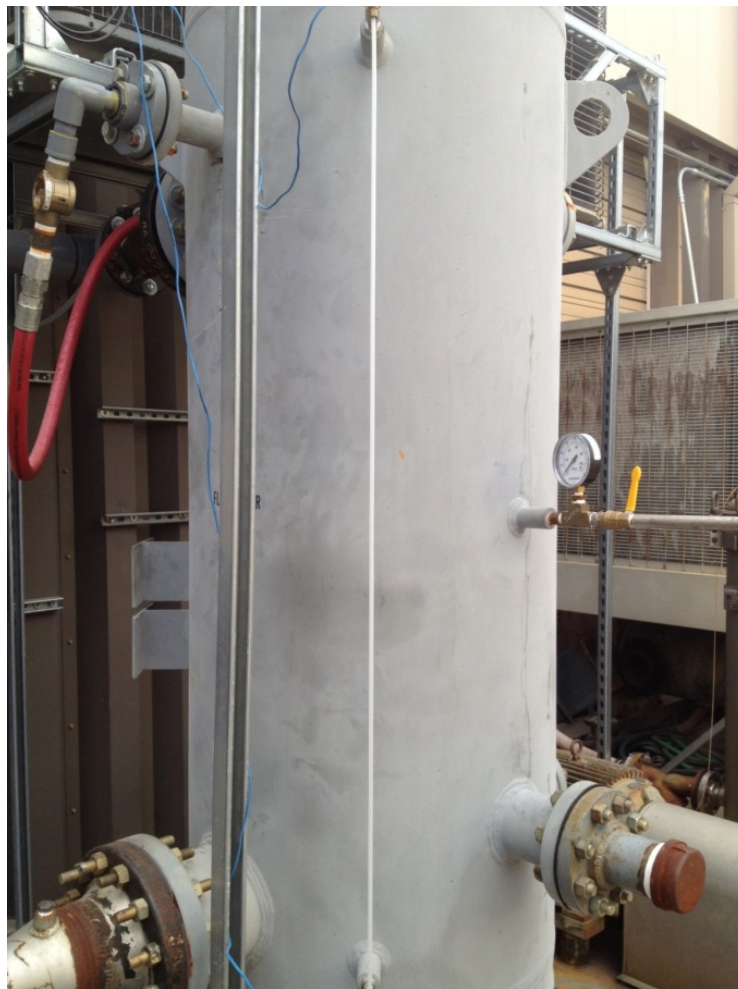
Figure 5: Water level indicator tube
