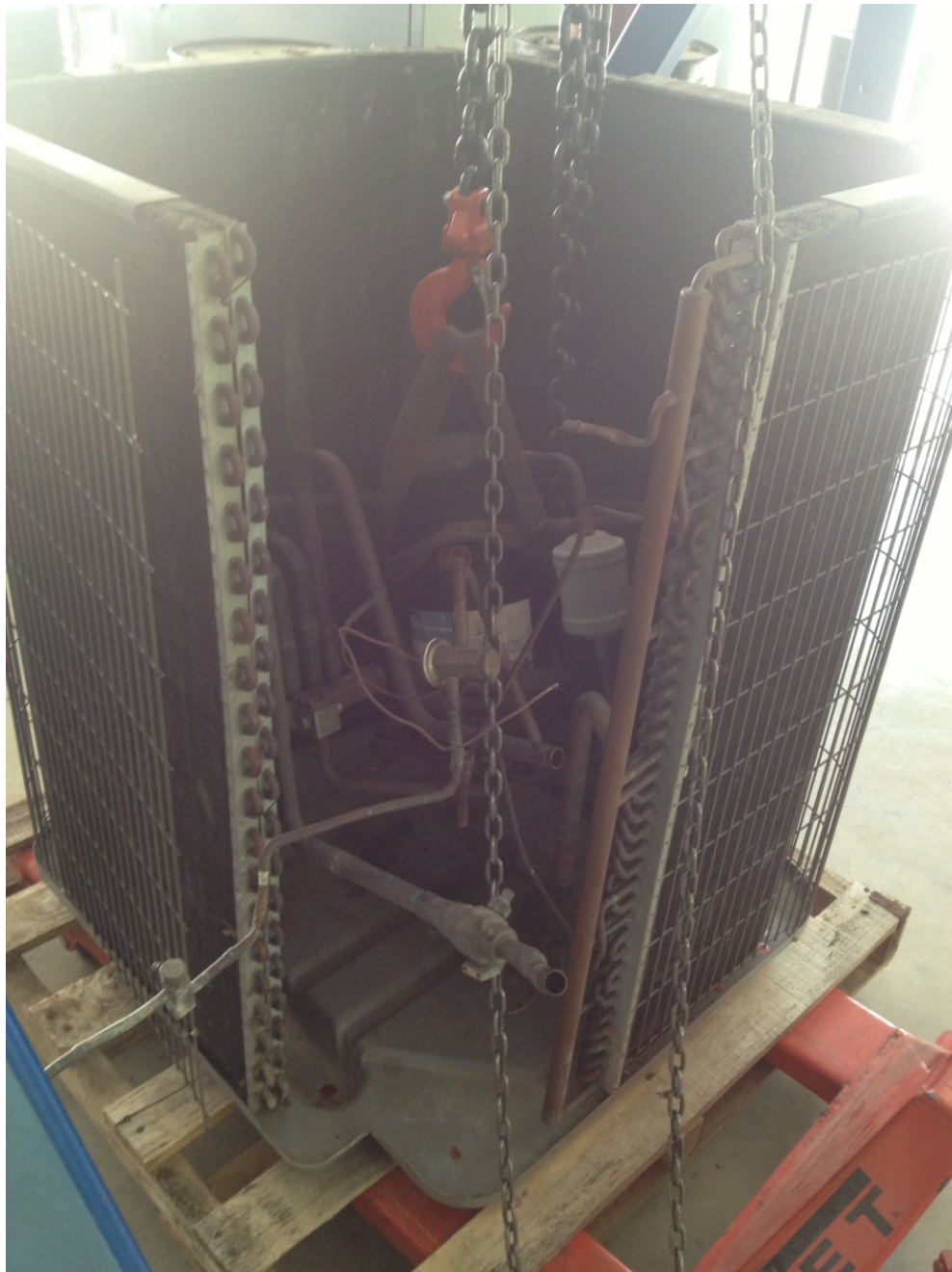
Figure 27: Compressor removal from HVAC unit
