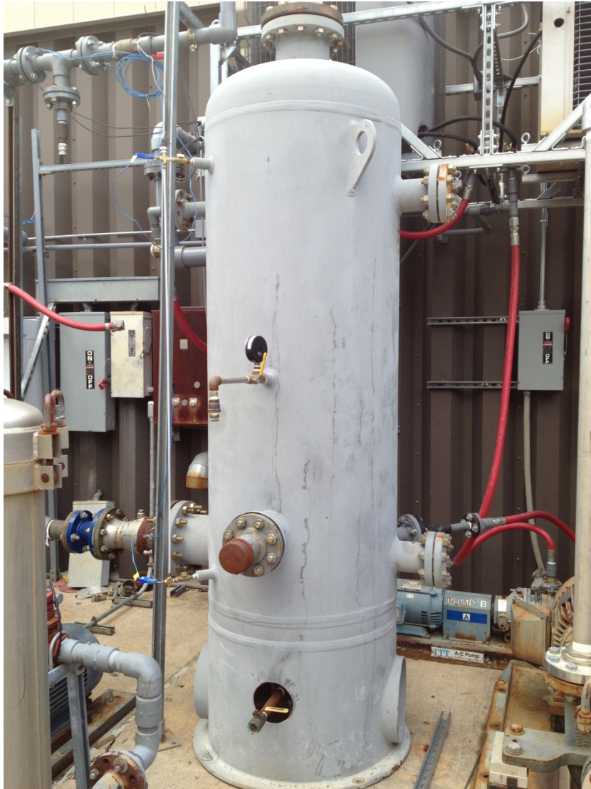
Figure 3: Gravity separator
