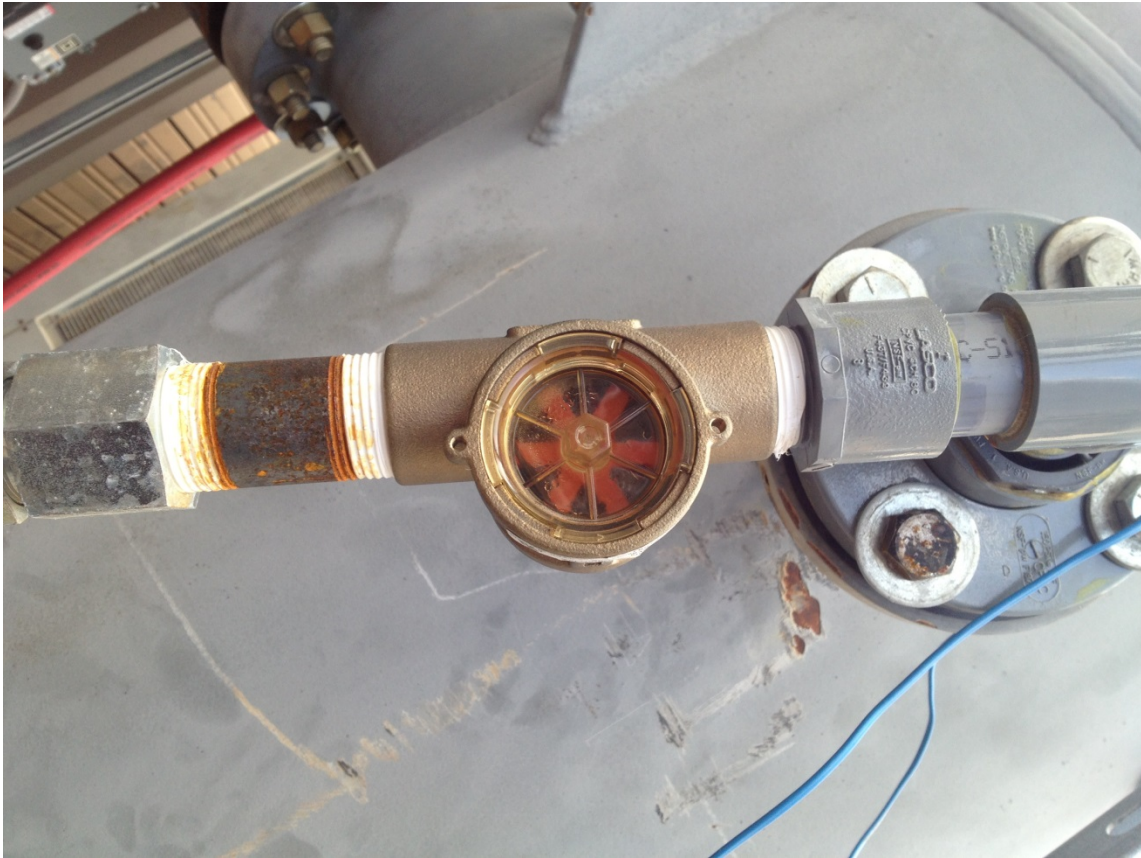
Figure 16: Rotary flow indicator
