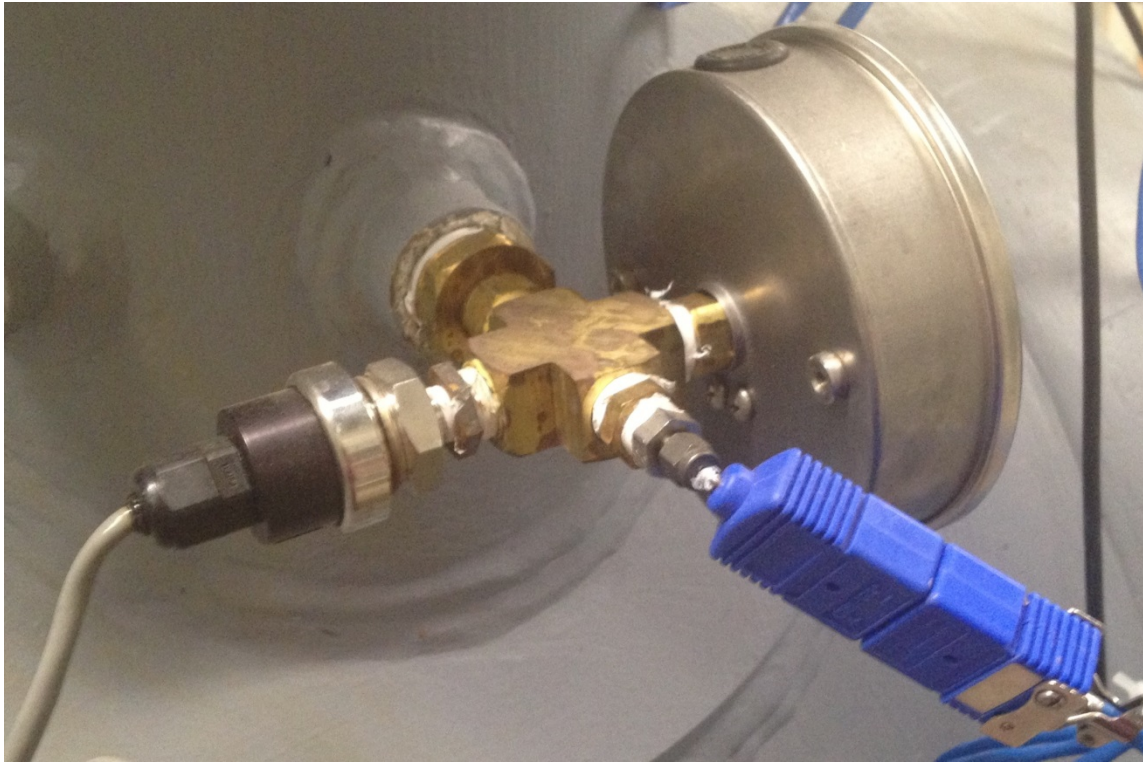
Figure 17: Pressure transducer at pump outlet
