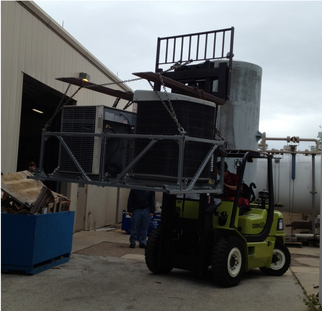
Figure 12: Heat exchangers and support structure being lifted into place
