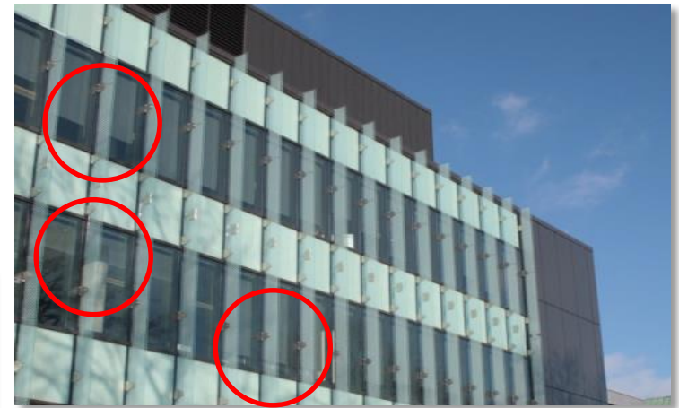
Figure 6 Blinds and side fins of the Genomics research center
