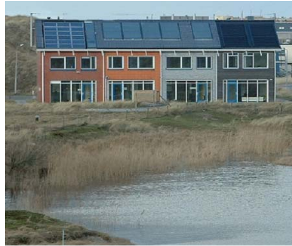
Figure 5: Above the four single family dwellings. The second house to the left is used for measurements with the adsorption chiller
