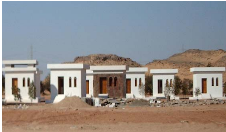
Figure 1. Photo for the test rooms in Toshky
