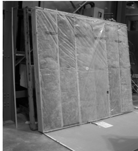
Figure 3 A poly-wrapped and unsealed (glass fiber) insulated wall.
