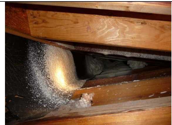
Figure 13 Beginning of north side sealing. (LaHiff)
