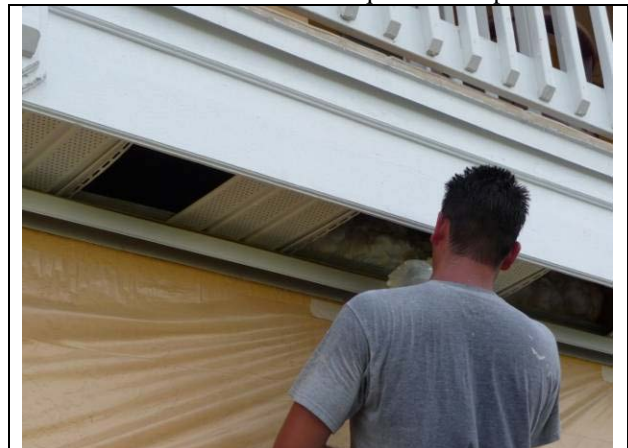
Figure 6 Foam application into west soffit area. (Withers)
