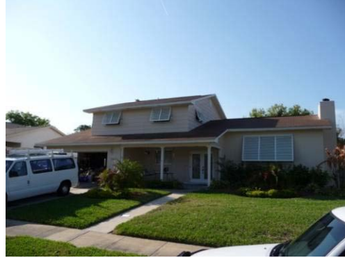
Figure 11 Front of split level home faces north. There is a small attic space above the front porch and garage which is open to the interstitial floor cavities.
