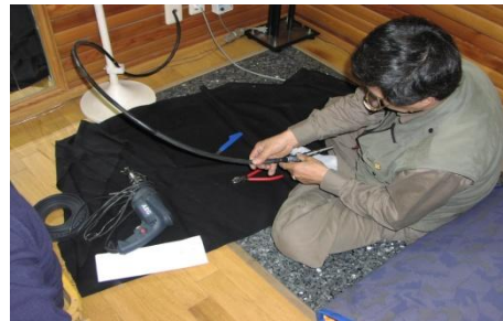
Fig. 11 Inspection of the status before repairing
