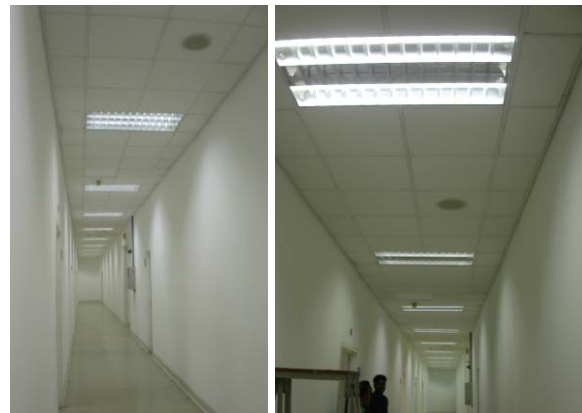
(a) (b) Figure 3. A corridor (a) before (b) after de-lamping
