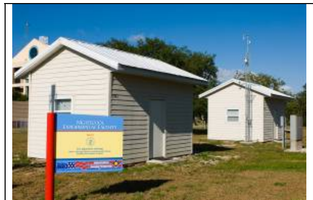
Figure 1. NightCool Building (left) and Control Building Under Test at FSEC
