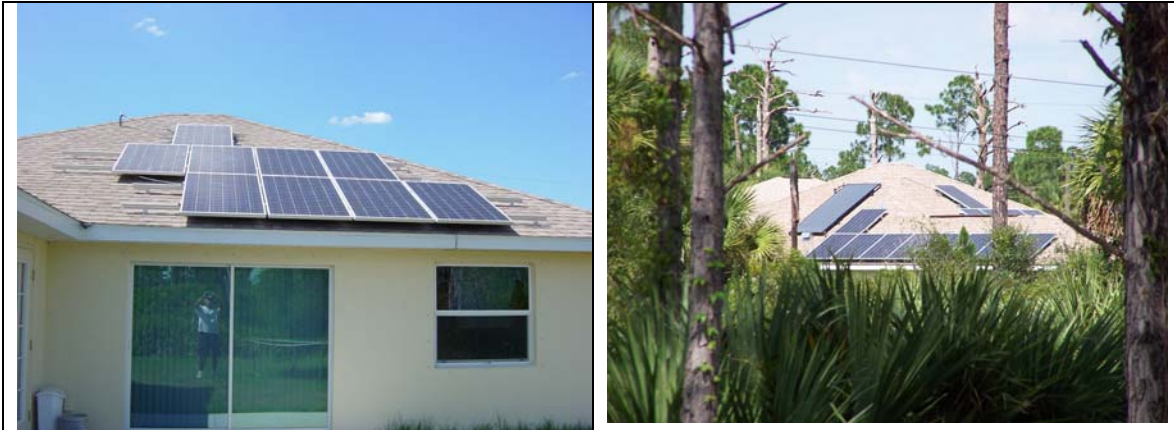
Figure 9. The Schroeders Homes NZEH in North Port, FL. The PV array is split on south and west roofs. Trees shade part of the array and the solar DHW collector in the afternoon
