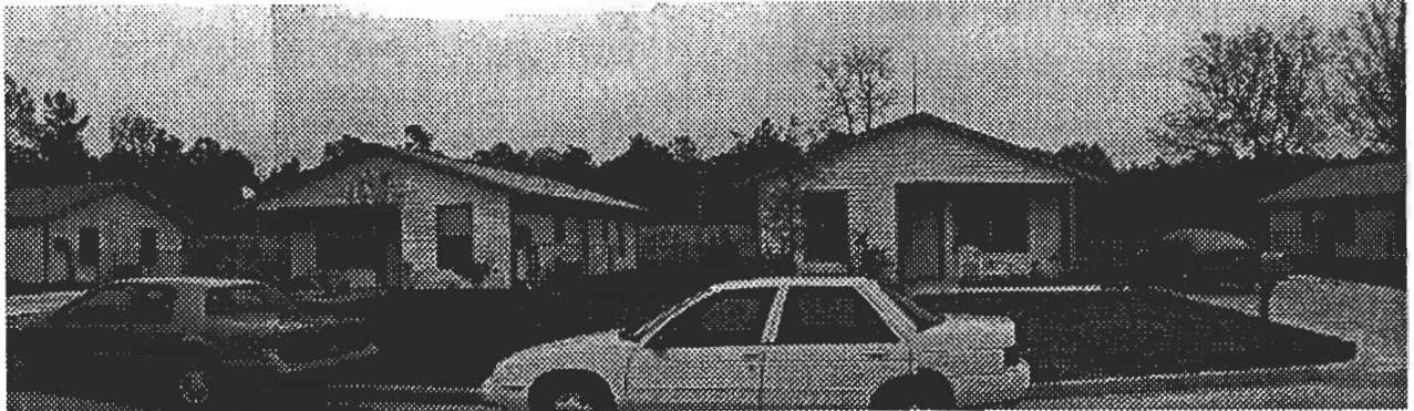
Figure 1. Front view of the two side-by-side Habitat for Humanity houses in Houston. The standard efficiency house is on the left and the energy efficient house is on the right.
