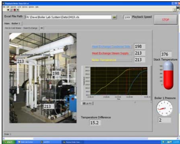
Fig. 8 Lab VIEW Boiler GUI
