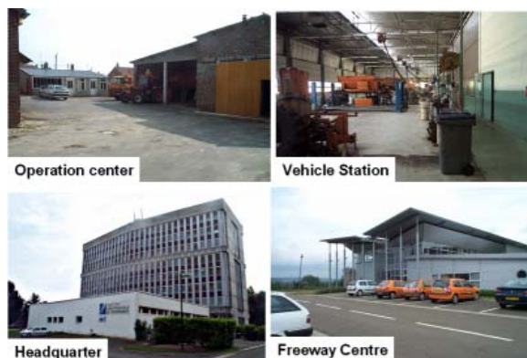
Figure 1. Photos of four types of buildings of the ministry
