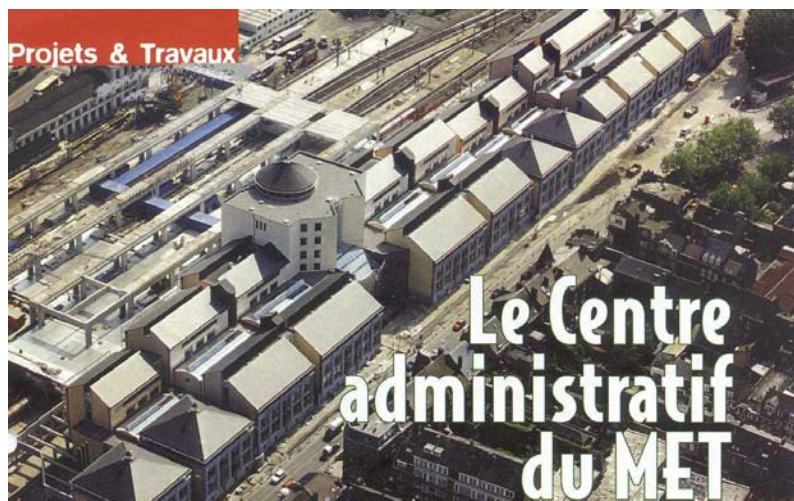
fig. 1 View of the « CA-MET » building
