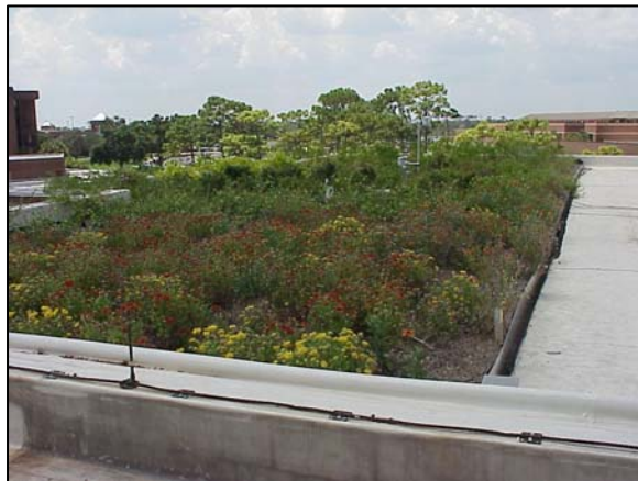
Figure 2. Green roof August 18th, 2005.
