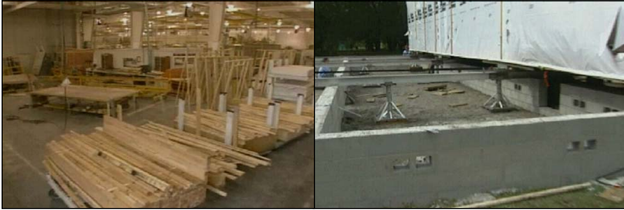
Figure 1. Manufactured and modular housing production facility (left). Prefabricated unit placement on concrete masonry unit (CMU) stem wall foundation (right) Jacobsen, 2005.
