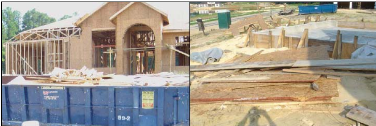
Figure 5. Typical site-built home construction site.
