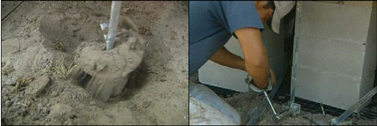
Figure 9. Galvanized auger anchors placed at a minimum depth of 1.2m (4ft) (left). Sidewall and frame ties spaced 1.6m (5.3ft) on center (right) Jacobsen, 2005.
