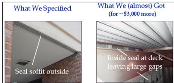
Figure 12. Specified vs. Contractor-planned Soffit Sealing Solutions
