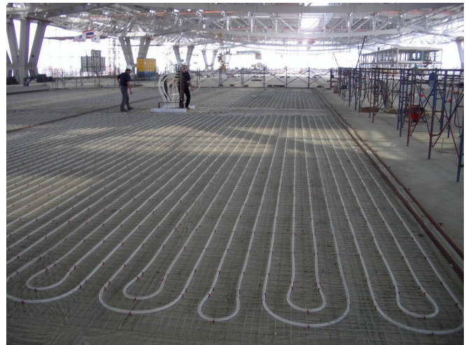
Figure 6 Radiant floor cooling system in construction
