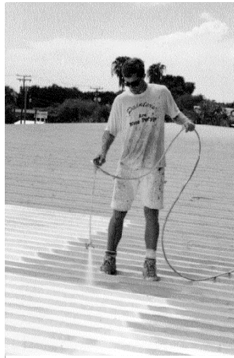
Figure 3. Phase II on roof whitening on July 30, 1997.
