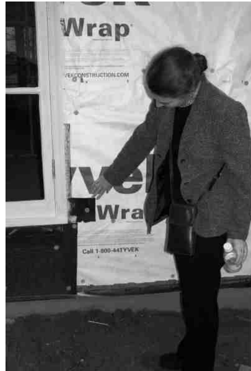
Figure 6a and 6b: Gaps in flashing at round-top window head.
