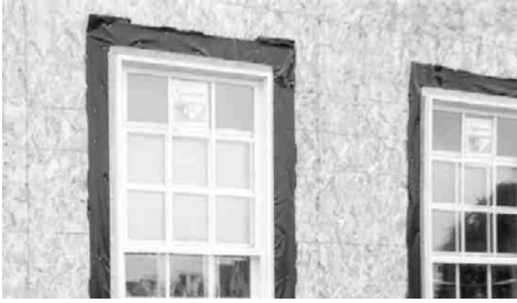
Figure 1: Reverse shingling at head flange.
