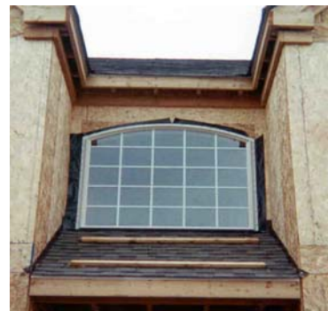
Figure 6a and 6b: Gaps in flashing at round-top window head.
