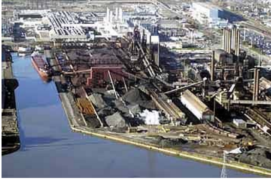
Figure 1: Ford's 1100 acre River Rouge industrial complex has a history of environmental degradation.
