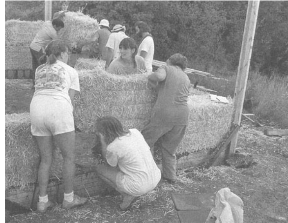
Figure 5: Straw bales lend themselves to unskilled labor and minimal tools.
