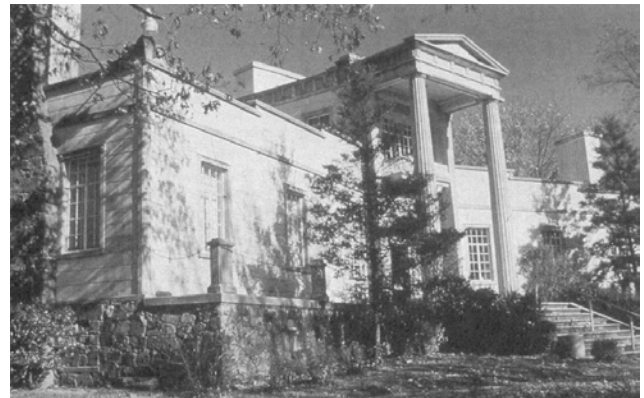
Figure 14: Exterior of Burritt mansion/museum, a two-story home built in 1938 in Huntsville, Alabama.
