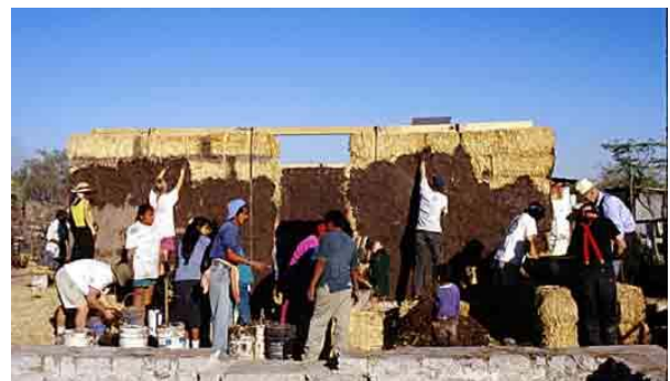
Figure 15: Community construction of the Canelo Project in Mexico.
