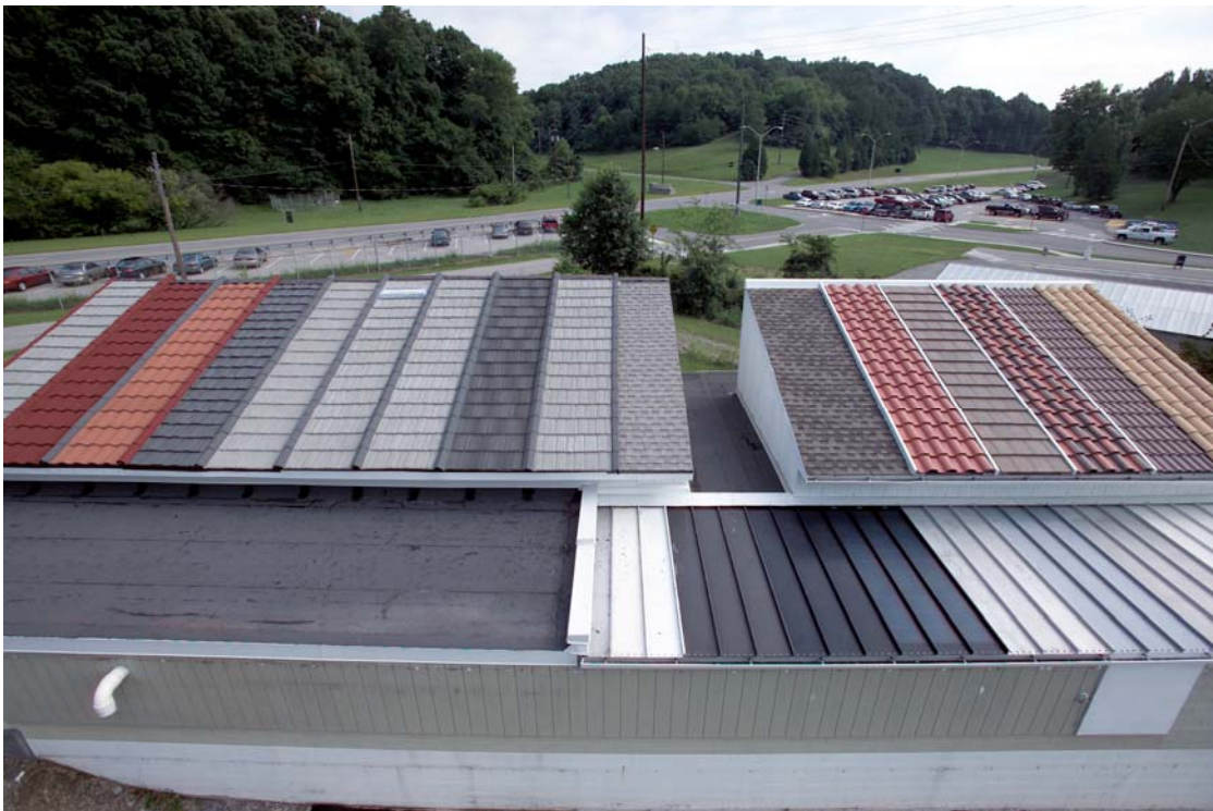
Figure 4. South-facing steep-slope attic assemblies placed atop the roof testing facility.
