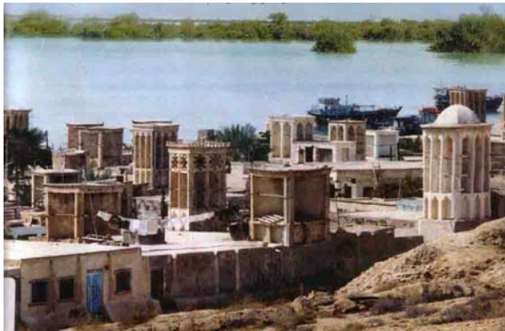
Figure 8- Wind towers of hot and humid region are usually larger than the ones in hot and arid region.
