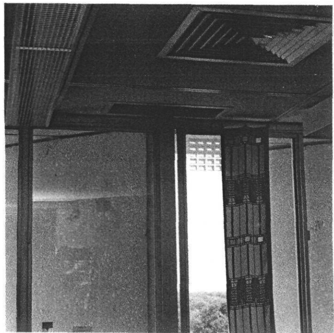
FIGURE 3. REFLECTORS USED IN AN OFFICE IN BUILDING A
