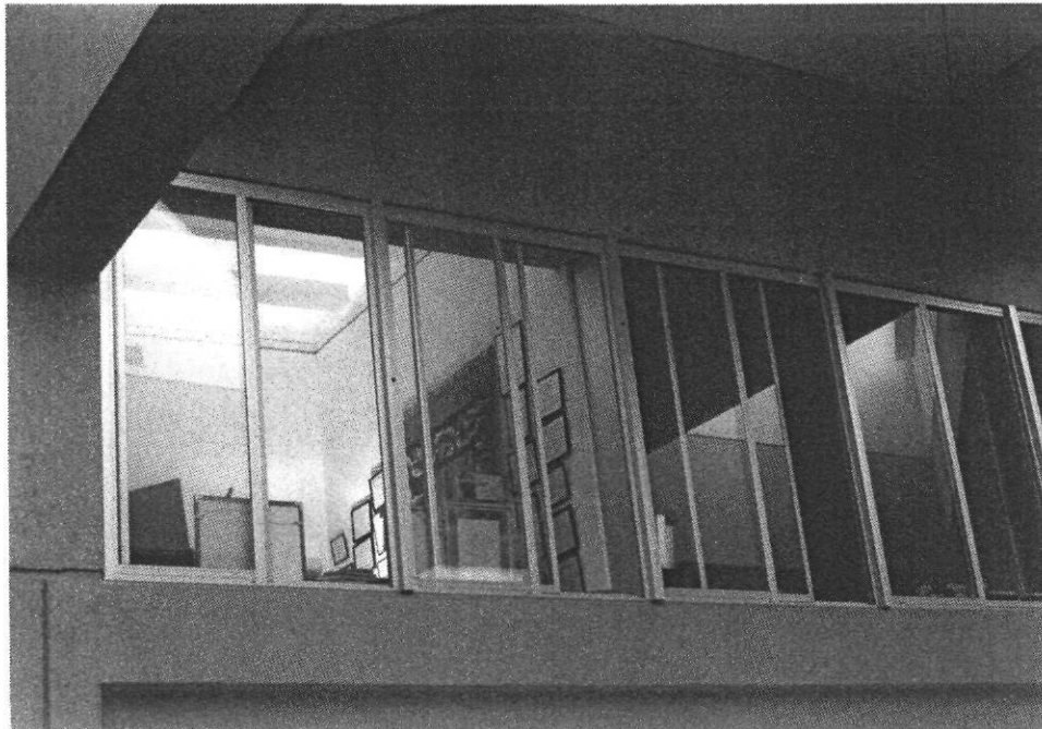
FIGURE 4. THE LIGHT “LEAKING OUT” TO THE ATRIUM
