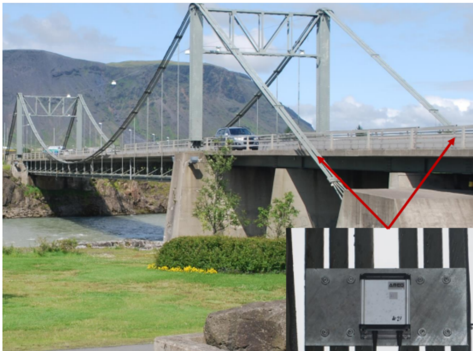
Figure 3.7: Accelerometers positioning (VEGAGERDIN, 2014)
