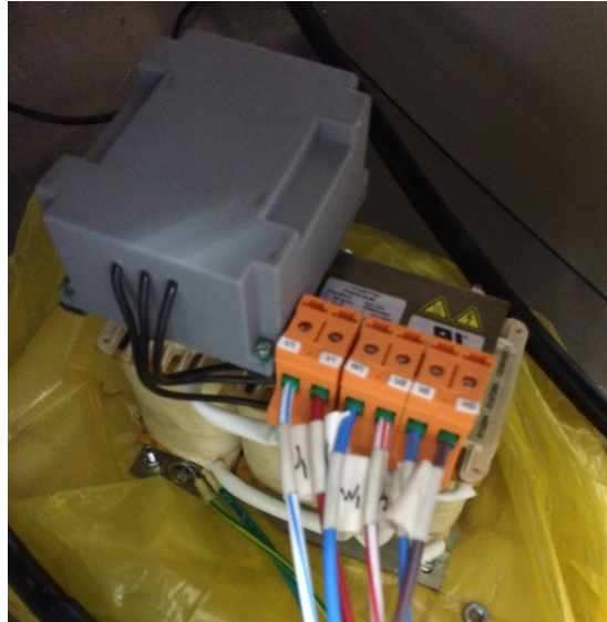
Figure 3.21 Sine filter by FN5040-24-84 Schaffner
