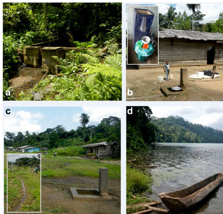
Fig. 3 Photographs of pertinent WASH infrastructures found at Barombi Mbo. a Gravity flow reservoir located 2 km away from the village. b Typical housing of Barombi Mbo with piped water stand nearby household grave [inset]. Sandbox water filter for household drinking water. c Village stand pipe for water; note open field drainage of water [inset]. Several open drains from piped water coalesce in the center of the village and form an open drain, as yet not colonised by snails which are found downstream: B. forskalii are found at site A5 (see Fig. 4c). d Lakeshore canoe landing site where many B. truncatus were found often in discarded cut bamboo and plastic containers amongst the water lilies and aquatic vegetation
