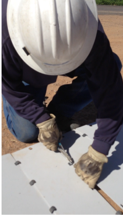
Figure 1.3.1 Guard's Slat Adjustment
