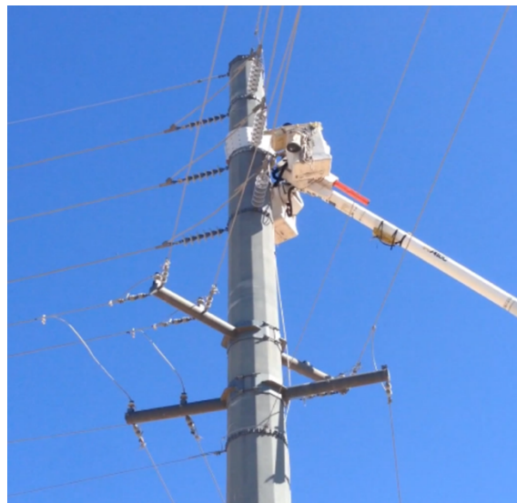
Figure 1.3.2 Raptor Guard Installation
