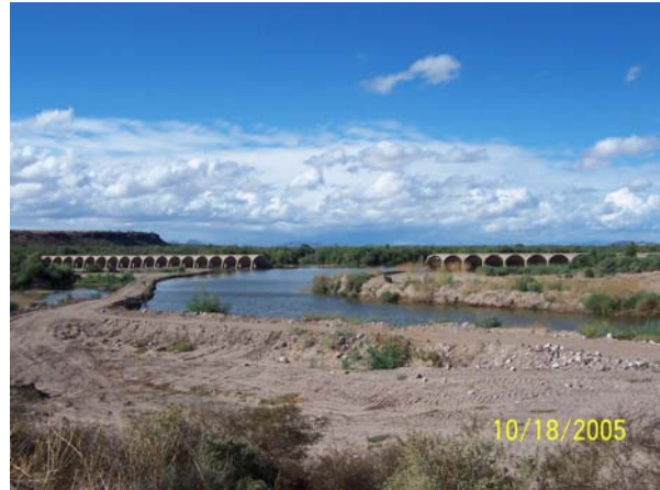
Looking north from Old U.S. 80 Bridge to Gillespie Dam
