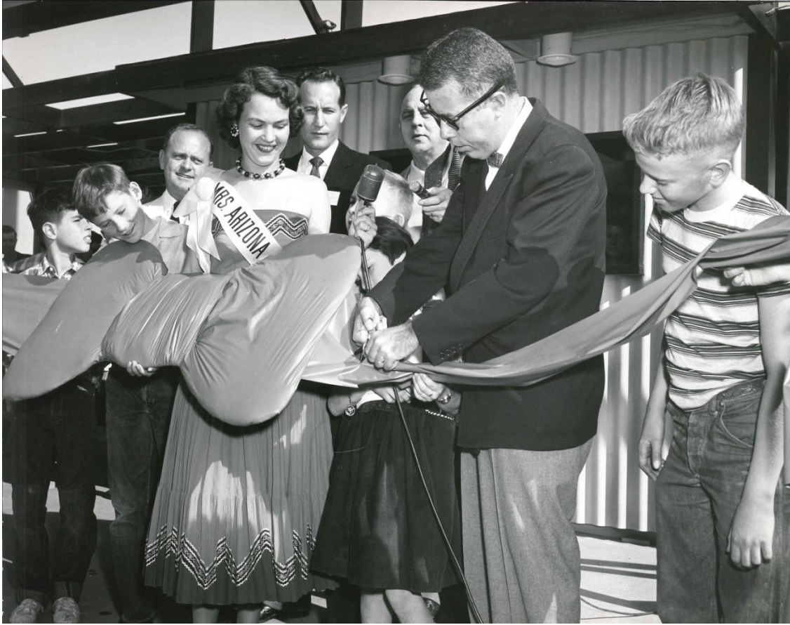
Figure 43: Ground Breaking Ceremonies, Parade of Homes, by Phoenix Association of Home Builders, Royal Crest Villa, 7 th Street and Hayward Avenue, Phoenix Arizona. Photographed by Bob Markow, (Courtesy: Arizona Historical Society, Home Builders Association of Central Arizona Collection: 1997), 1956.
