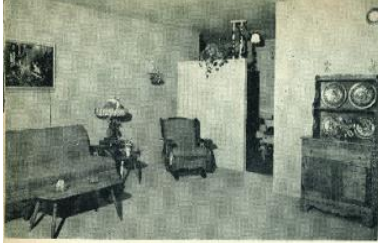
Living room of the "Maryvale Terrace" home has tasteful wall finishes. One is exposed brick, another is a smooth, colored finish, and the third, a wooden louvered divider which provides a decorative feature for the room.
