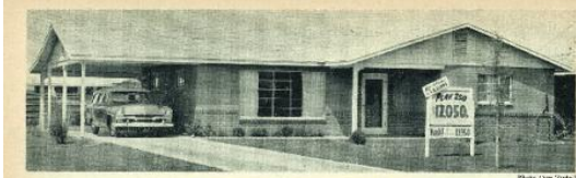
"Highland Estates" homes are built of brick at the bottom with Superflex garage blocks above, topped with a composition roof. Lot sizes are 70-80 x 110.
