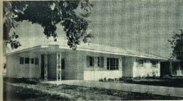
White pull-cock ports lend charm to this home's exterior. Built of sturdy pumice block, contrasting color shingles are added for style.
