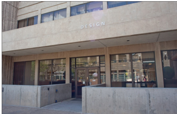
Figure 26: Altered signage above the building's entrance
