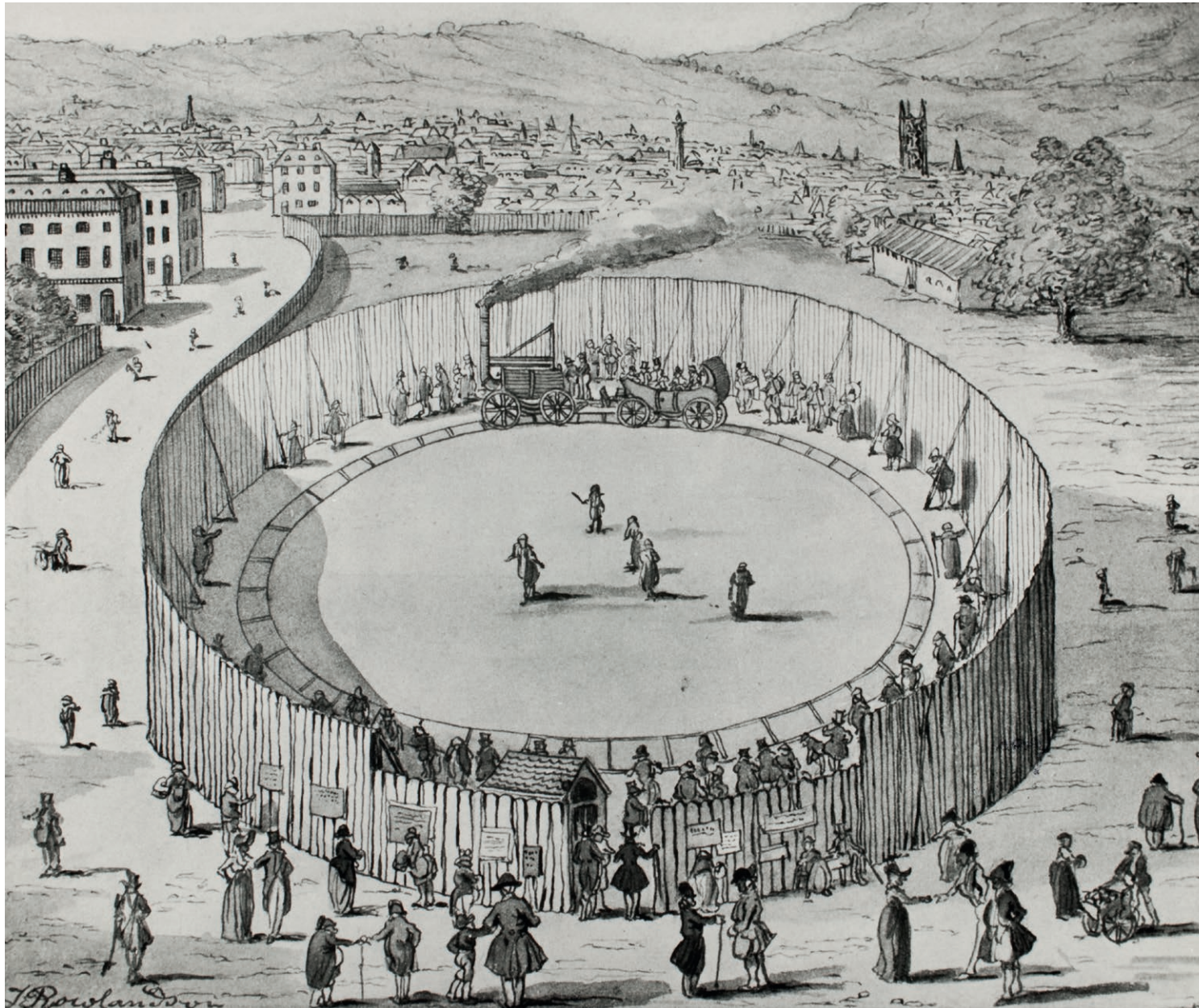
In 1808 the engineer Richard Trevithick demonstrated a steam locomotive called Catch-me-who-can on a site near the top of Gower Street, the future site of UCL. It was the first experimental passenger railway powered by steam. (Cartoon ascribed to Thomas Rowlandson, copy held in UCL College Archive: Photographs)
