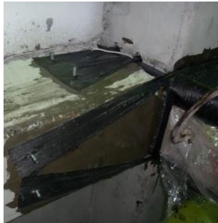
Step 6: Strengthening of beams and joint with FRP strands
