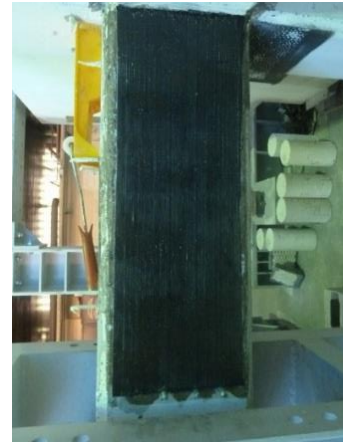
Step 7: Application of strips of FRP for shear strengthening and anchorage in beams; additional anchorage with bolted steel plates
