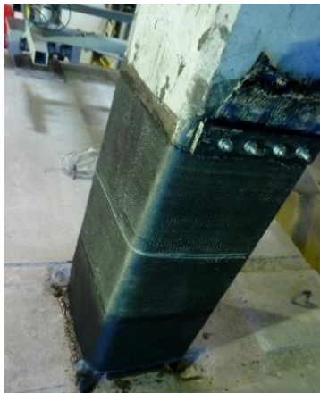
Step 5: Column confinement and shear strengthening
