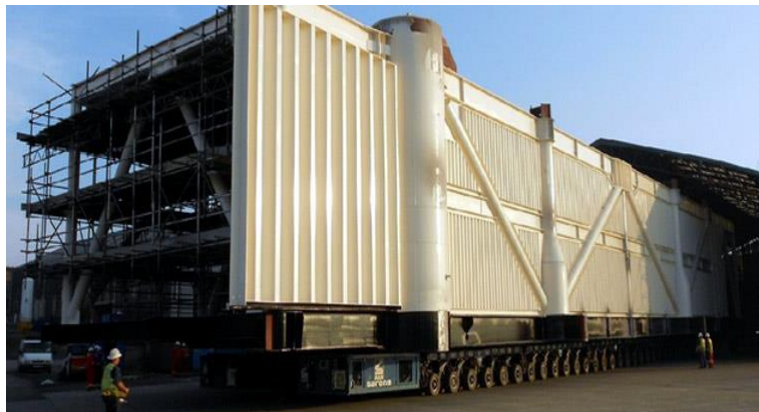
Figure 2. Typical blast walls on offshore installations (Mech-Tool Korea, 2014).
