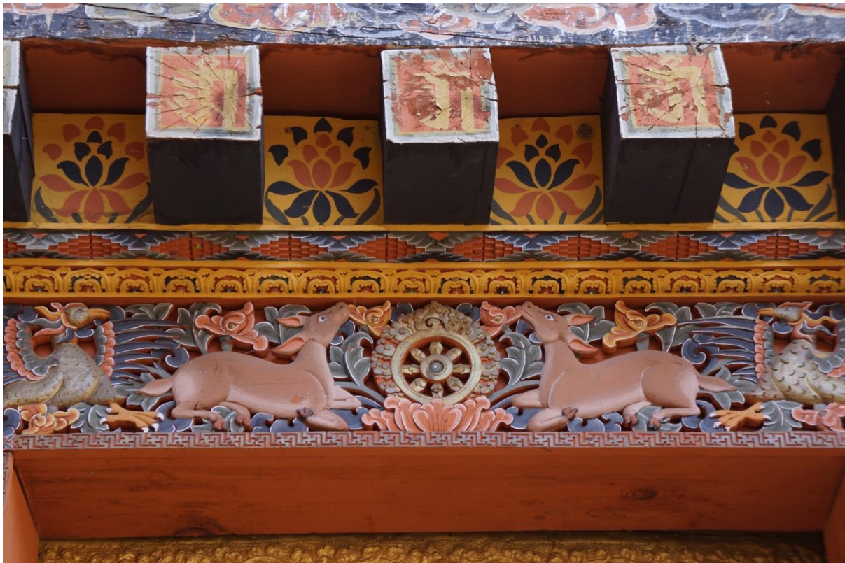
Figure 16. Complex carved and painted woodwork. Conserving this represents a major challenge in terms of maintaining traditional craft skills in timber preparation, carving and painting.
