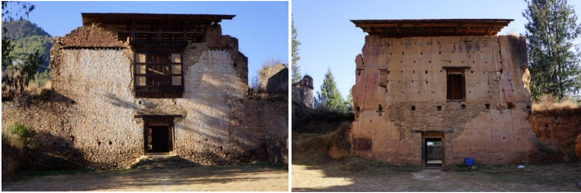
Figure 23. Outer gatehouse: exterior (left) and interior (right), with temporary roof.
