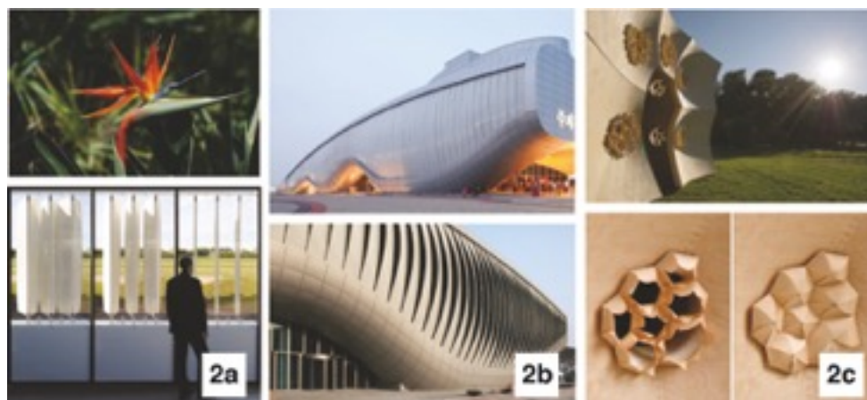
Figure 2. Examples of biomimetic projects for adaptive architectural envelopes: (a) Flectofin® (b) One Ocean Thematic Pavilion (c) HygroSkin
